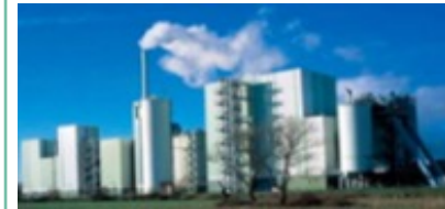
Waste Incineration Plants
