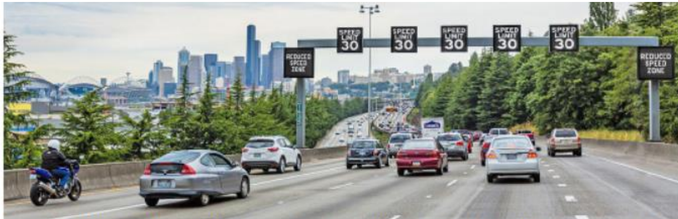
Figure 2. Photo. Variable message signs showing traffic alerts and speed limits for individual lanes.
