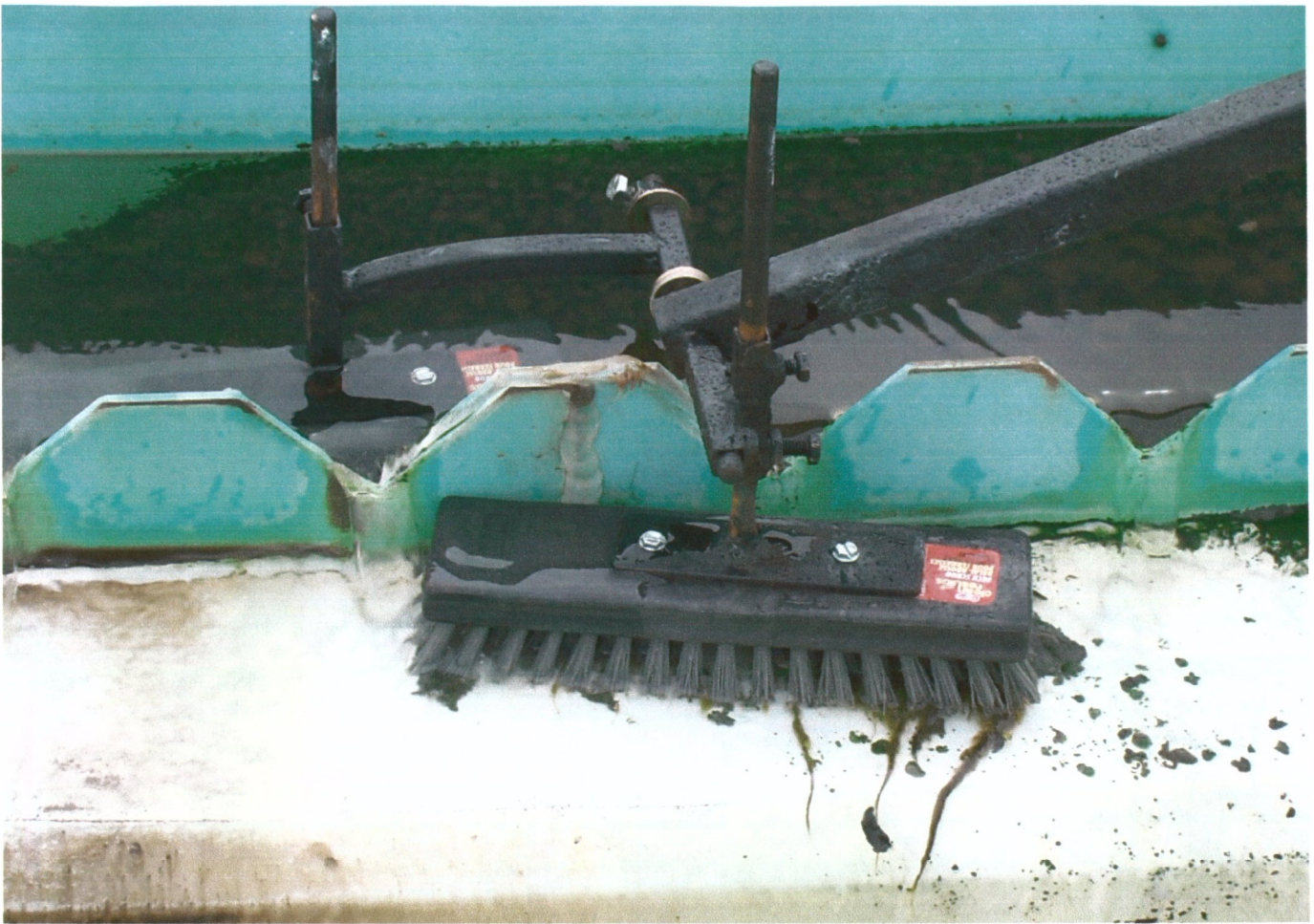
Replaced brushes and painted arms and altered inner brush mount.
