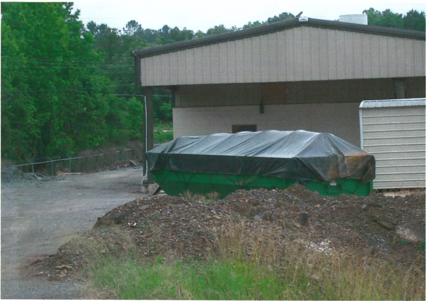
Tarp over dumpster with bows installed.
