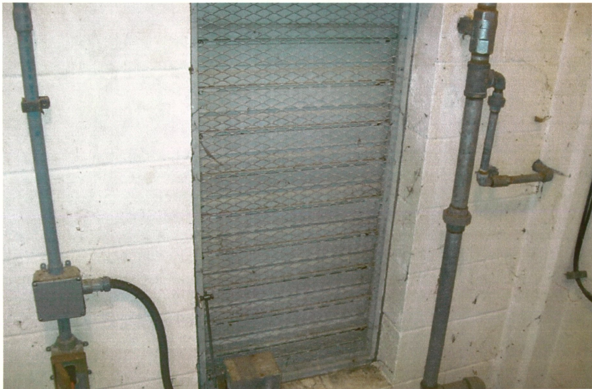
Repaired vent in SO2 room.
