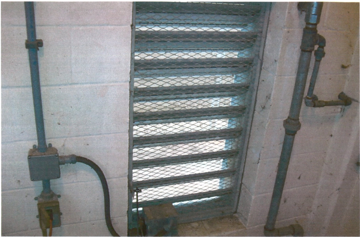
Repaired vent in SO2 room.
