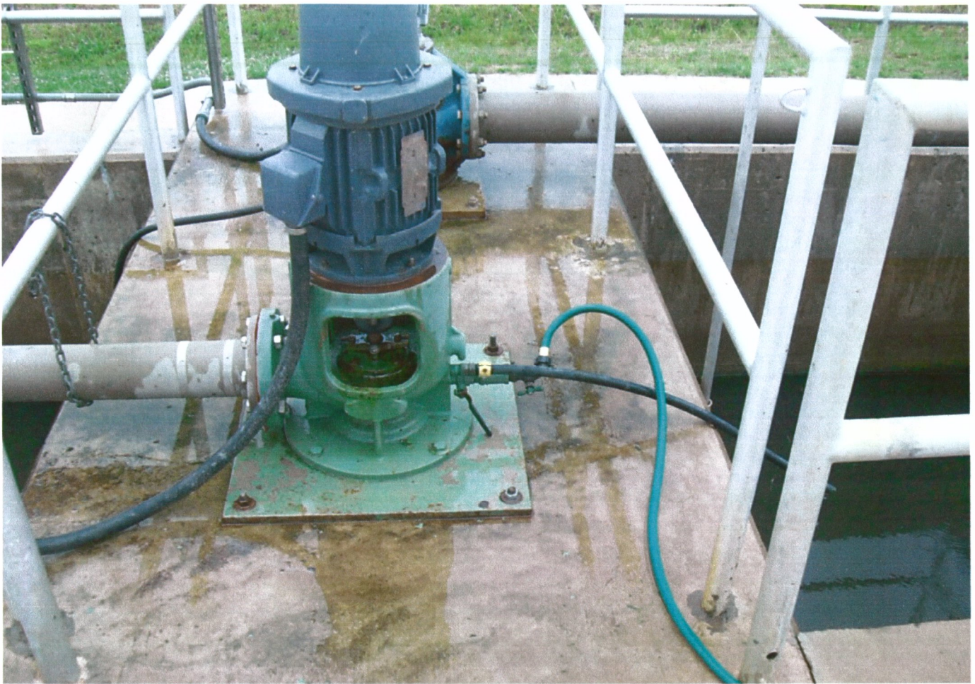
Replaced seals in makeup water pump.
