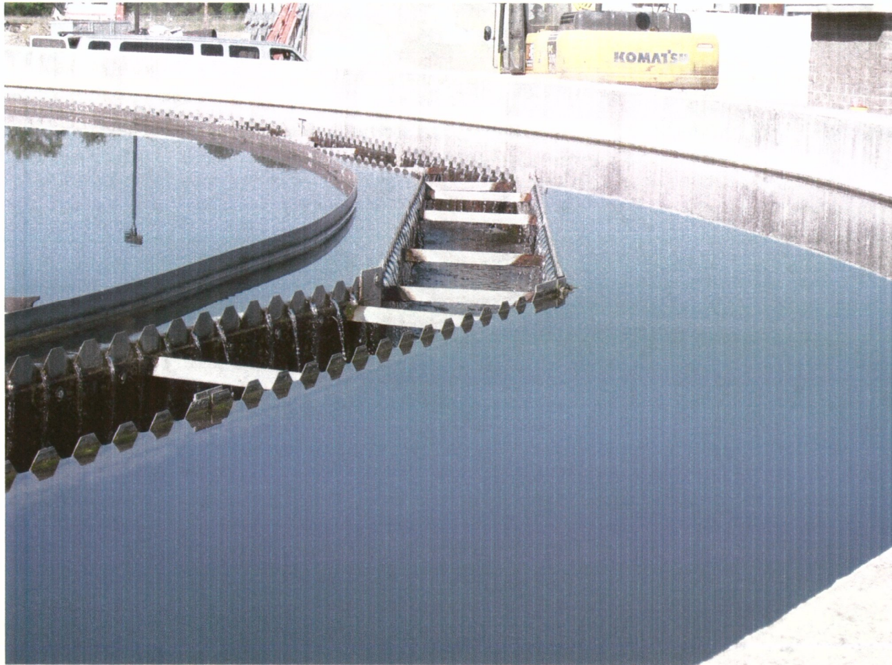
Issue 1. A. #2 Clarifier - weirs & baffles cleaned.
