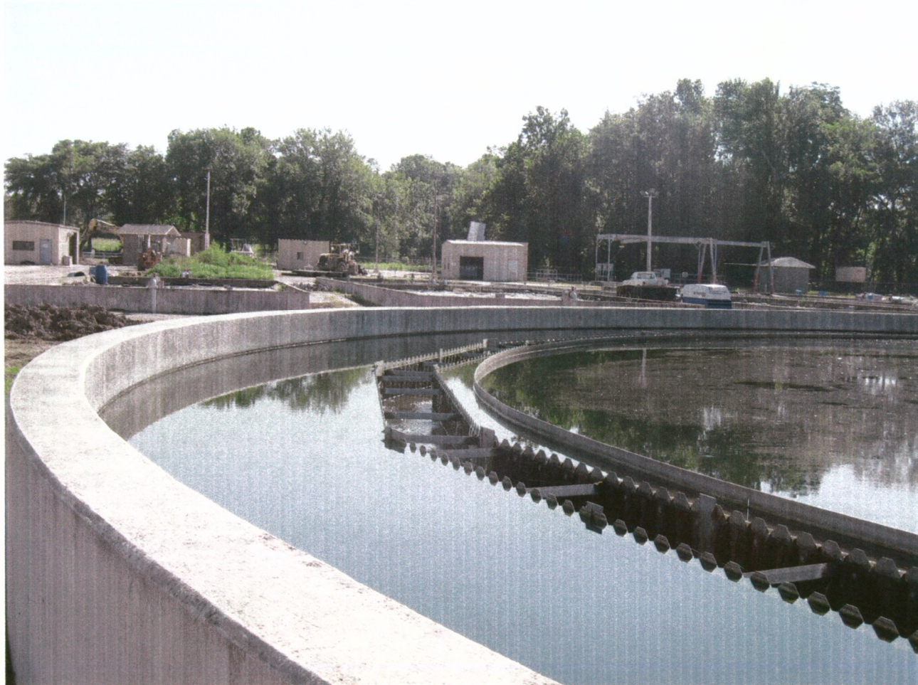
Issue 1. A. #1 Clarifier - weirs & baffles cleaned
