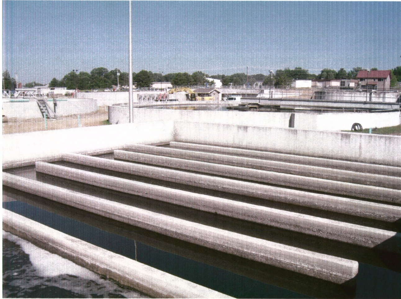
Issue 1. B. Chlorine Contact Chamber no floatables.
