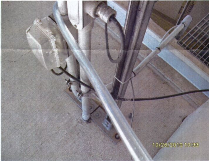
Sampler Tubing Replaced
