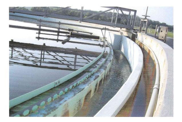
Picture of secondary weirs with better chlorine flow. With the addition of a booster pump Garver is working on, all the weirs should get an even dose of chlorinated water.
