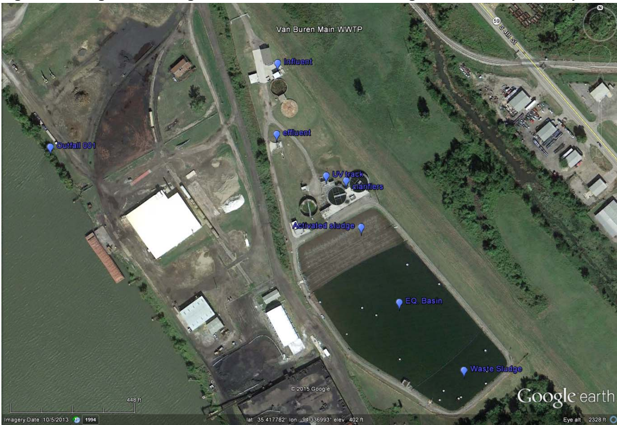
Figure 1: Google Earth image dated October 5, 2013 showing overview of treatment plant.
