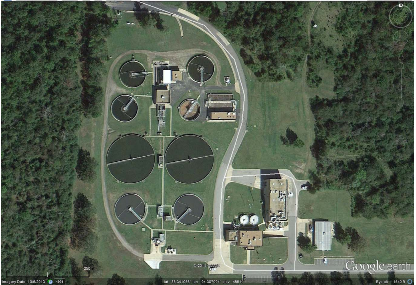
Figure 1: Google Earth image dated Oct 5, 2013 showing Massard WWTP overview.
