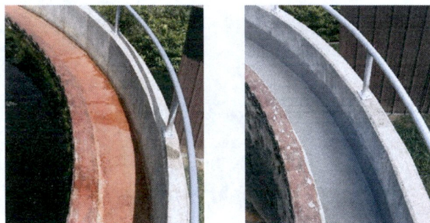
Gravity Thickener Tank Launderer – Before and After Repair, Respectively
