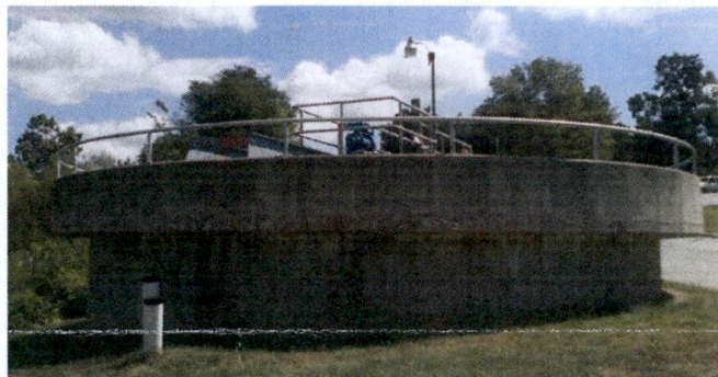
Gravity Thickener Tank – Repaired and In Service
