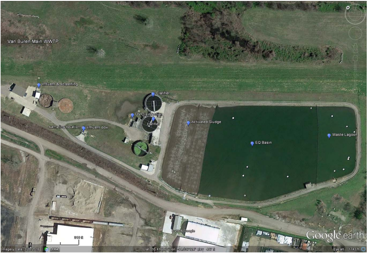
Figure 1. Google Earth image dated March 20, 2016 showing overview of treatment plant and major components.
