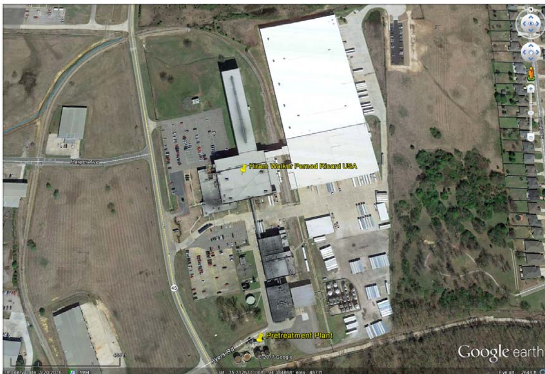
Figure 1. Google Earth image dated March 20, 2016 showing facility overview and pretreatment plant location.
