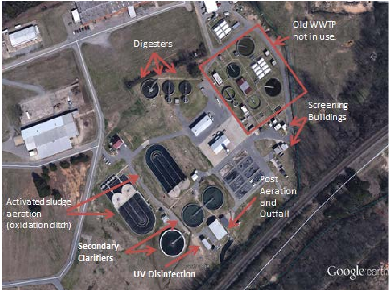
Figure 1: Overview of Benton wastewater facility.
