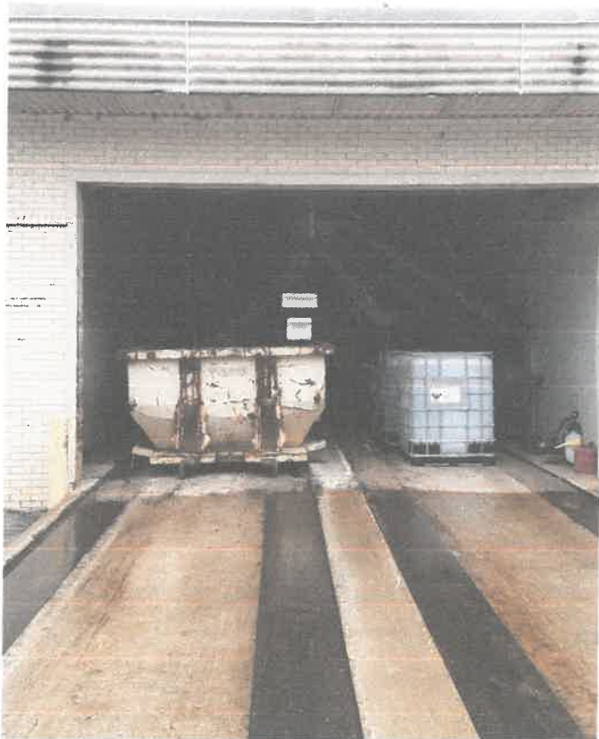
Picture 9 Totes Stored in Building with drain capture system.
