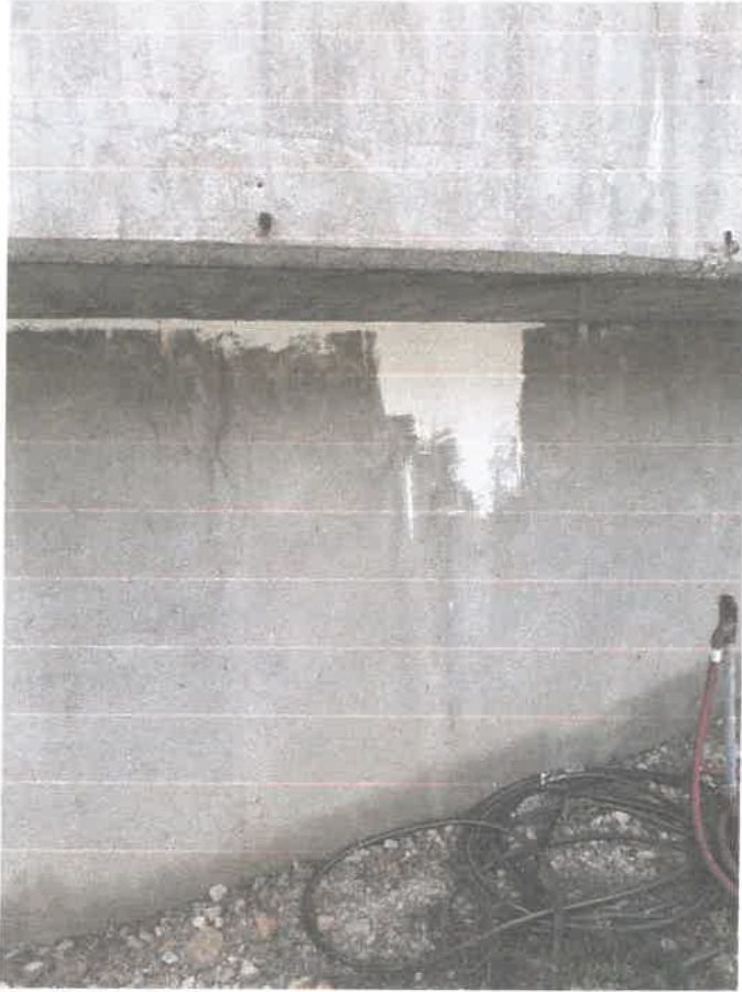
Picture 3 Primary Clarifier 1 Repair Photo
