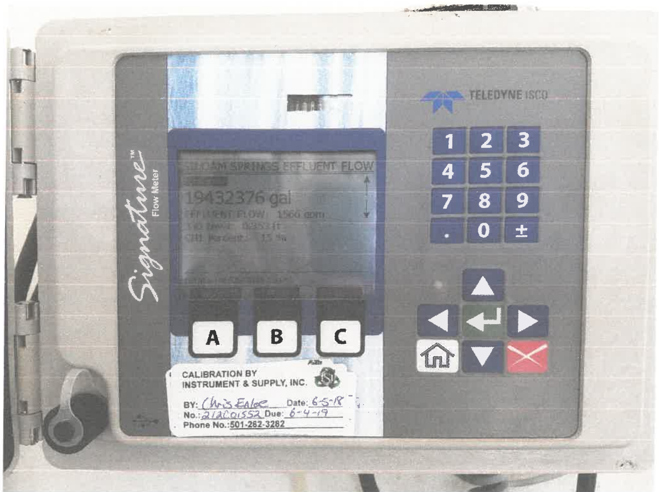
Picture 6 New Inspection Certification.
