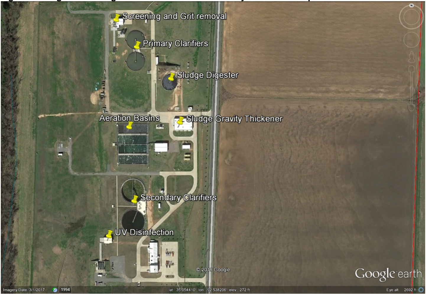
Figure 2. Google Earth image dated March 2017 with facility treatment components noted.
