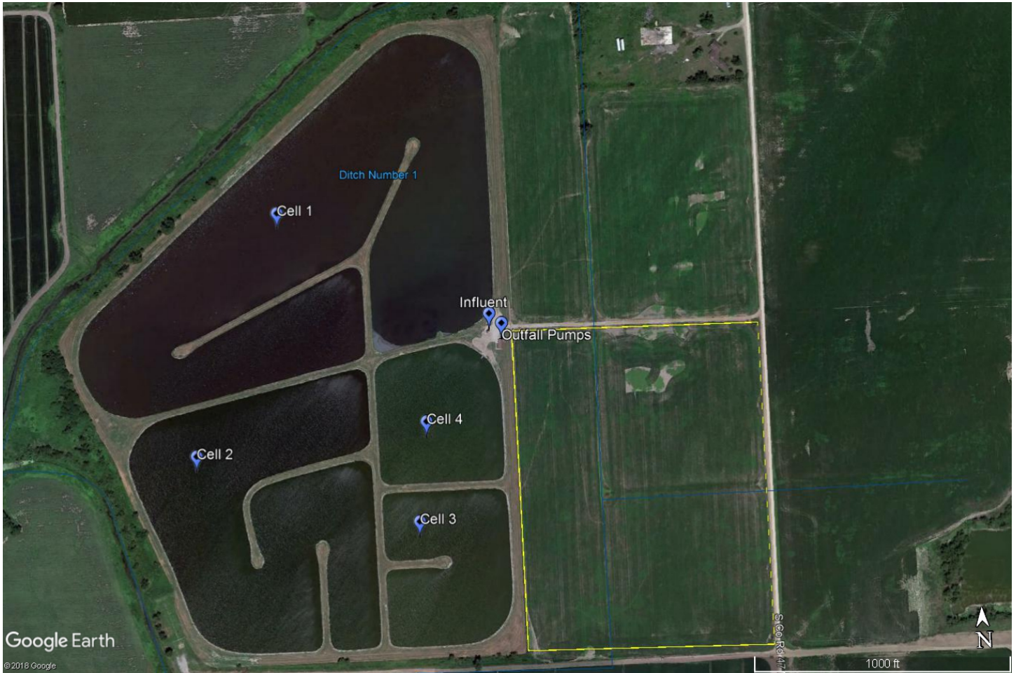
Figure 1. Google Earth image of the Osceola WWTP with labels for the different portions of treatment. Note the square area identifying the construction site for the additional cells.
