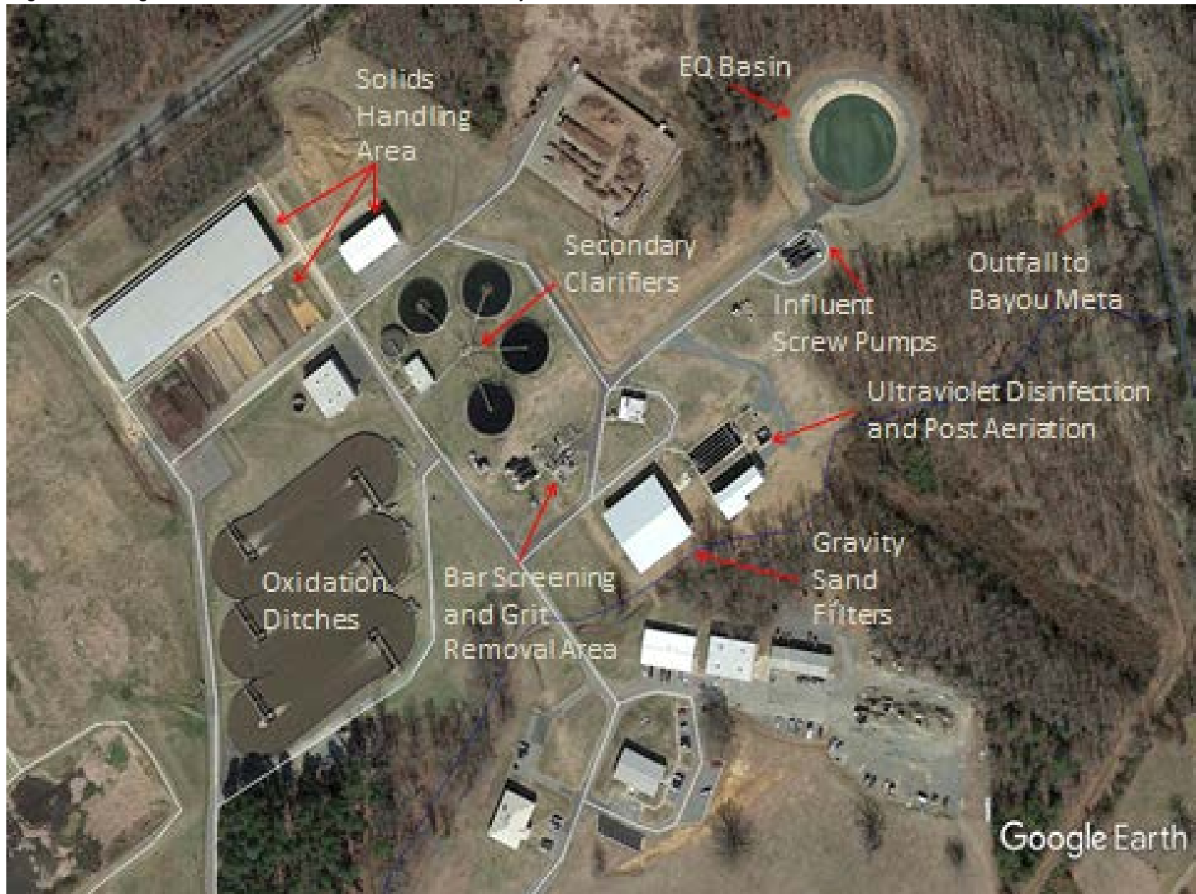
Figure 1: Google Earth Image of Jacksonville wastewater treatment facility.
