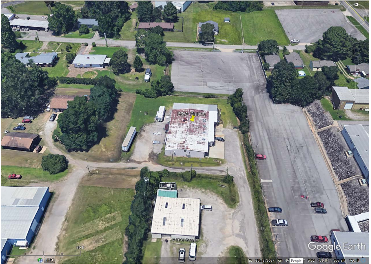
Figure 1. Google Earth image dated May 31, 2019 showing facility overview.
