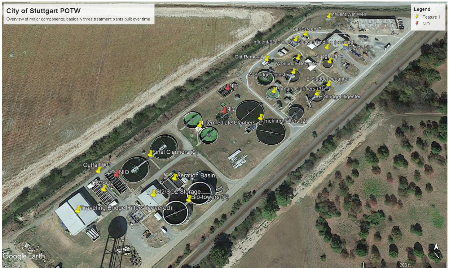
Figure 2. Google Earth image dated Oct 14, 2015 depicting the City of Stuttgart POTW with major components identified. Red pins are components that are not in operation (NIO).
