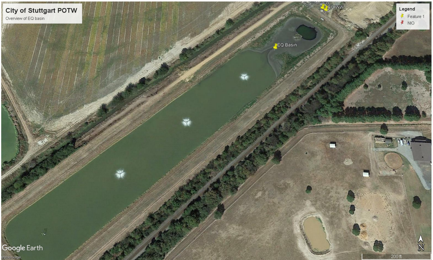
Figure 3. Google Earth image dated Oct 14, 2015 depicting the City of Stuttgart EQ basin with major components identified.
