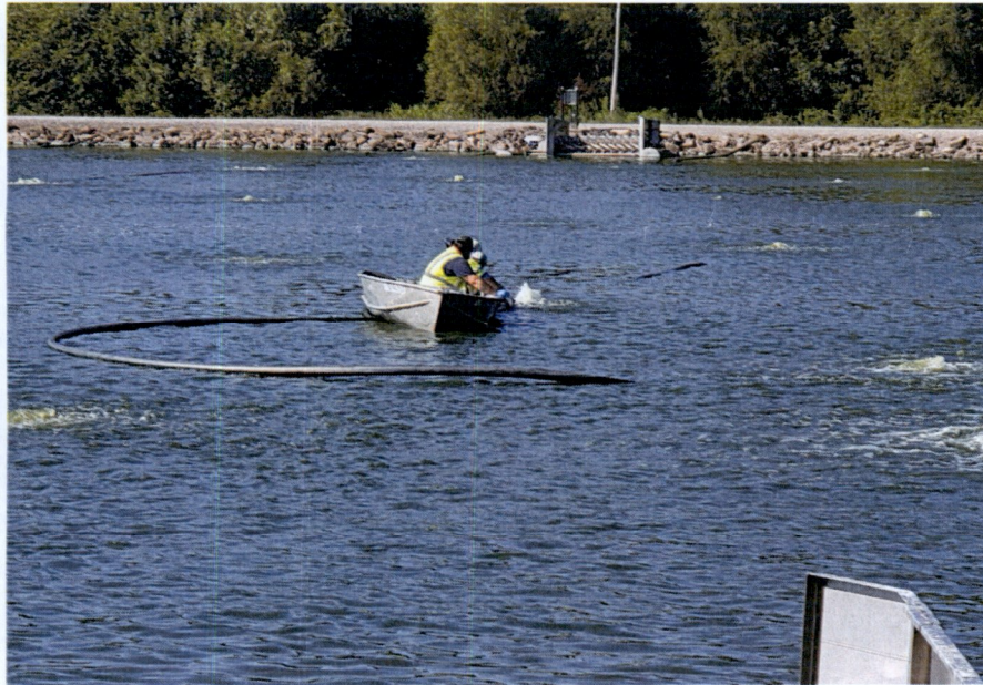
2 A. The crew repairing the broken airline in the lagoon. 8/18/20
