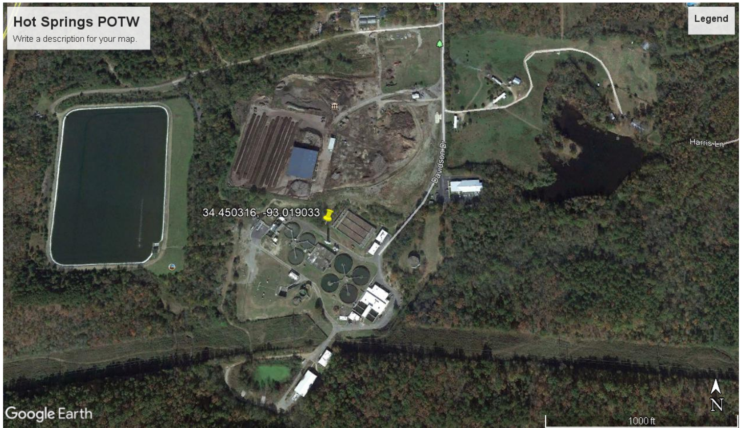
Figure 1. Google Earth image of City of Hot Springs POTW.
