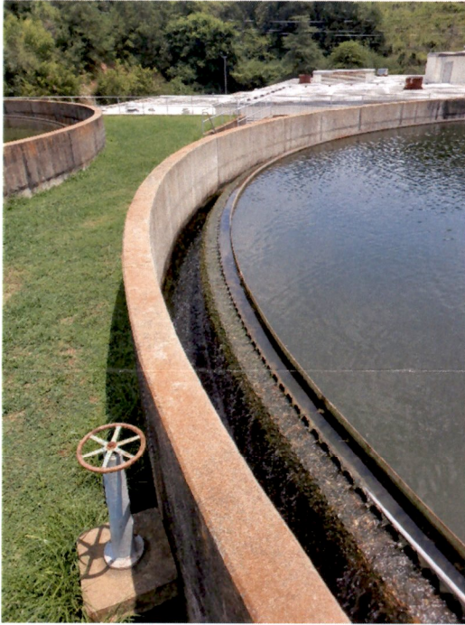
Clarifier after cleaning
