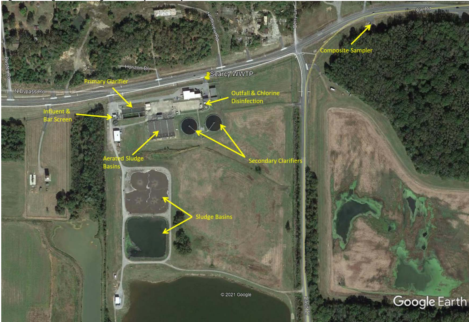
Figure 1: Google Earth image of the City of Searcy Wastewater Treatment Plant.
