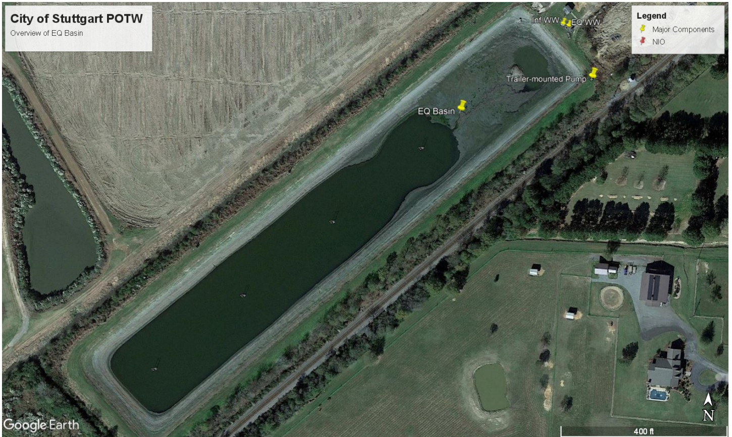
Figure 3. Google Earth image dated November 2020 depicting the City of Stuttgart EQ basin with major components identified.
