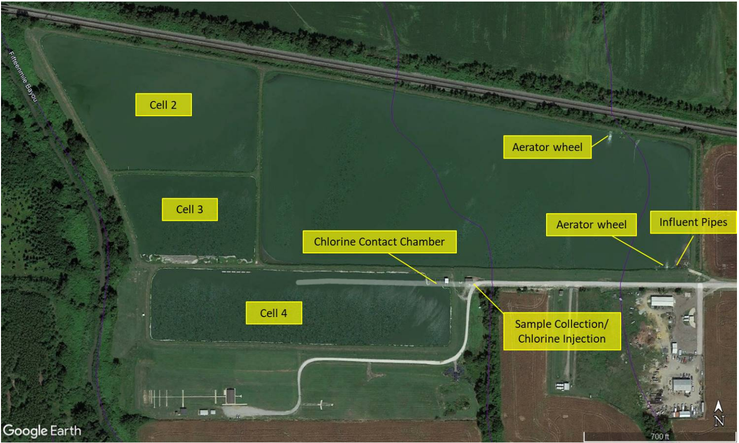
Figure 1. Google Earth image of the City of Marion POTW with labels for the different areas of treatment.
