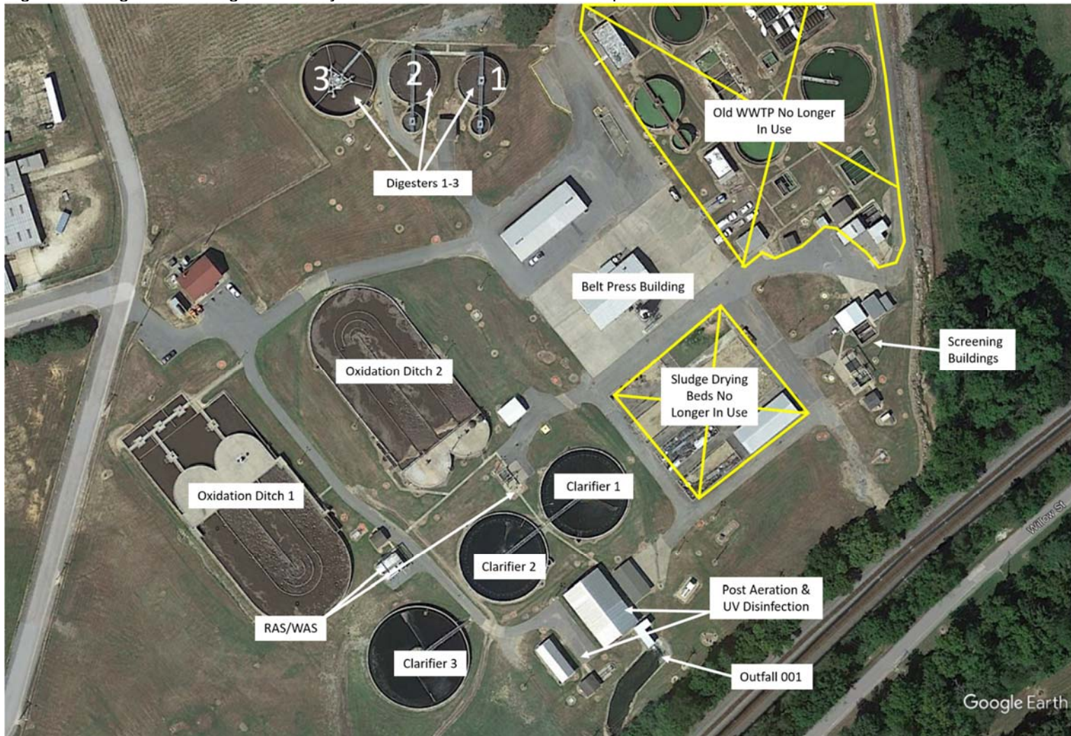
Figure 1: Google Earth image of the City of Benton wastewater treatment plant.
