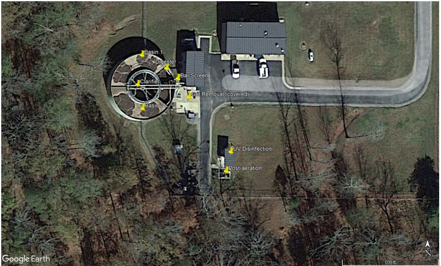
Figure 1. Google Earth image dated Nov 15, 2020 of the Southside Public Water Authority WWTP with major components labeled.
