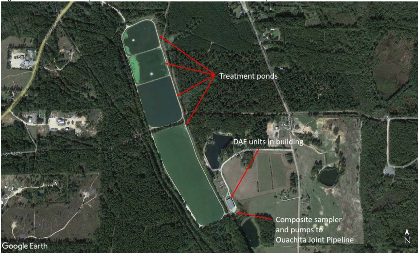
Figure 1. Overview of City of El Dorado – South Plant with the treatment components indicated.
