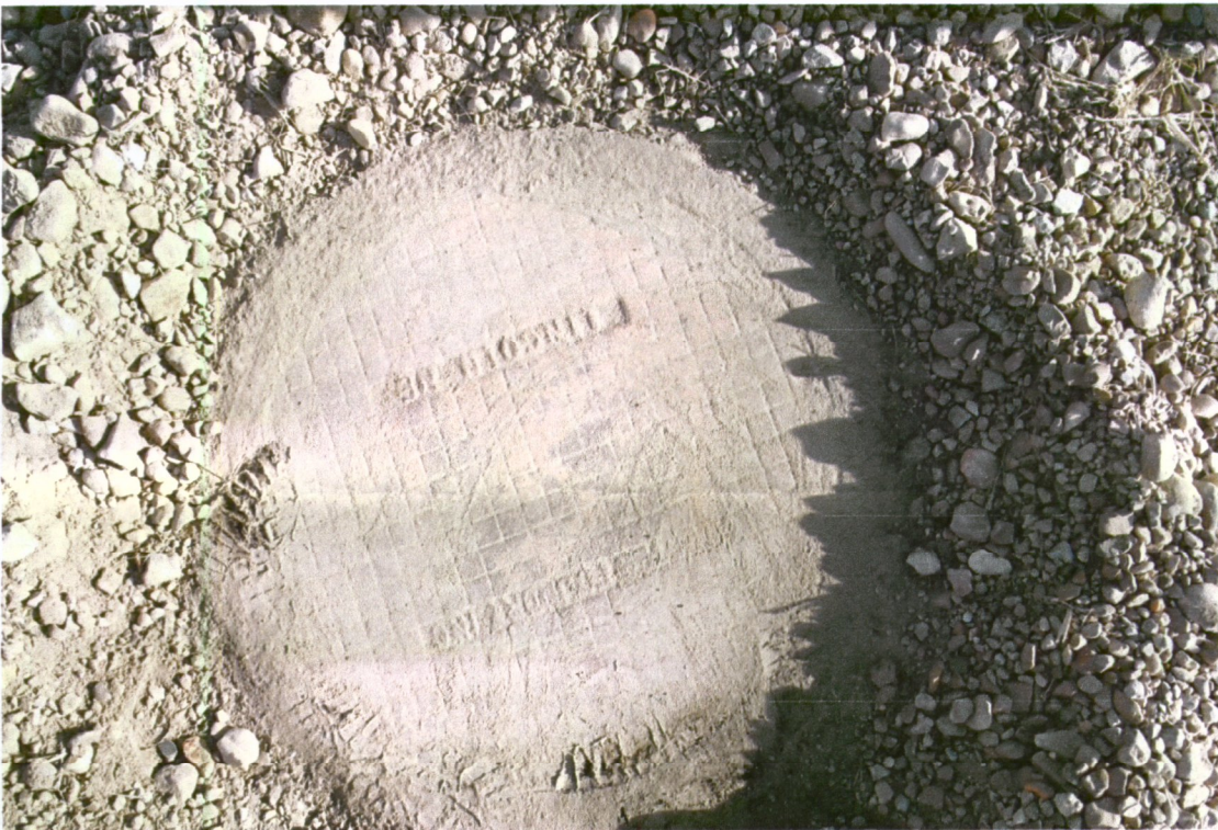
Manhole at Pump Station #3 (note grout ring has been replaced)
