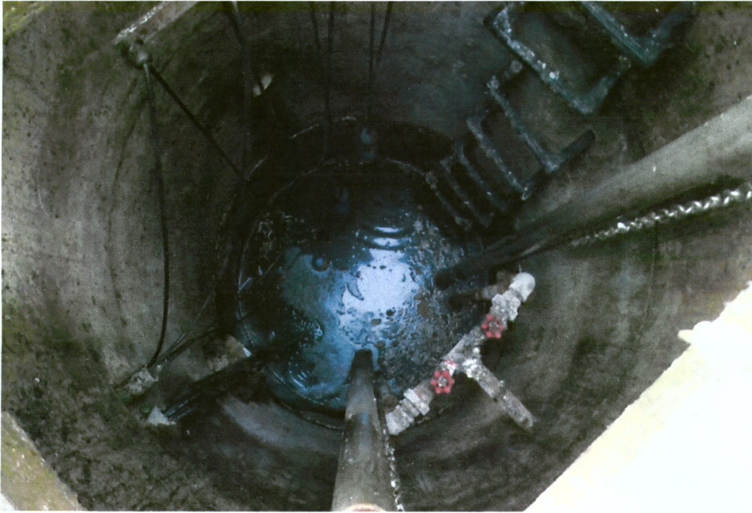
Pump Station #2 Interior
