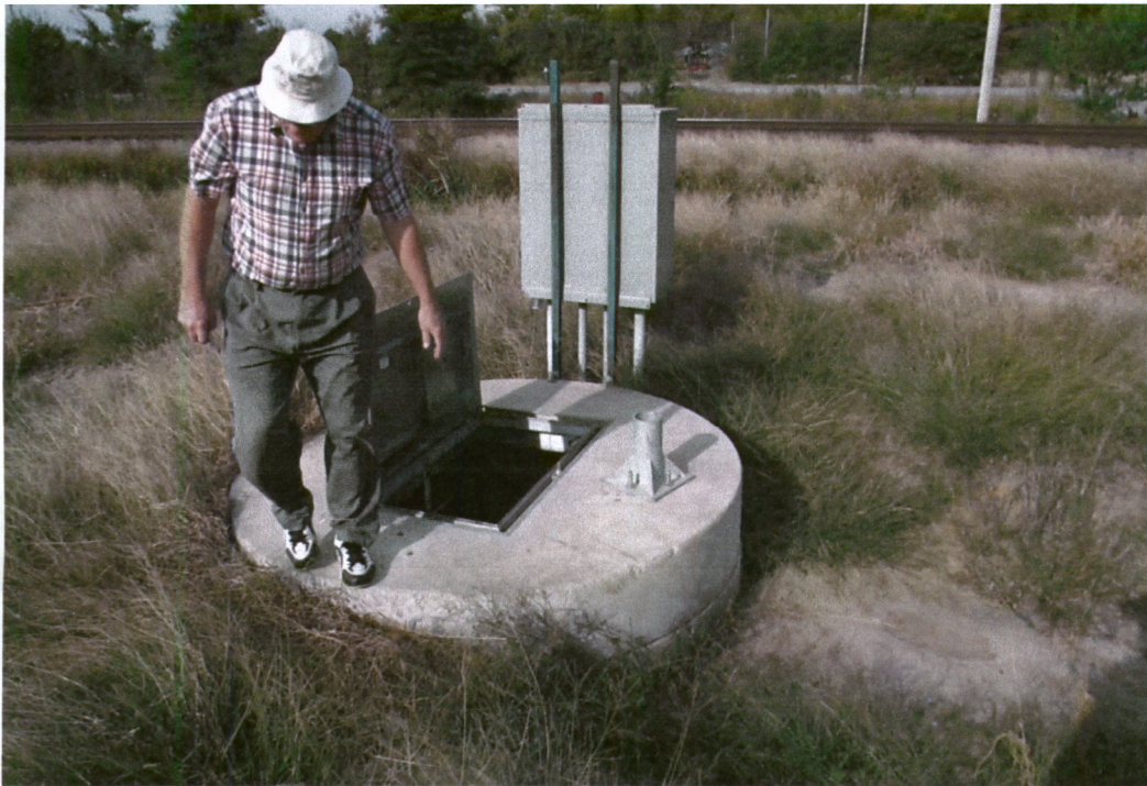
Pump Station #6 exterior
