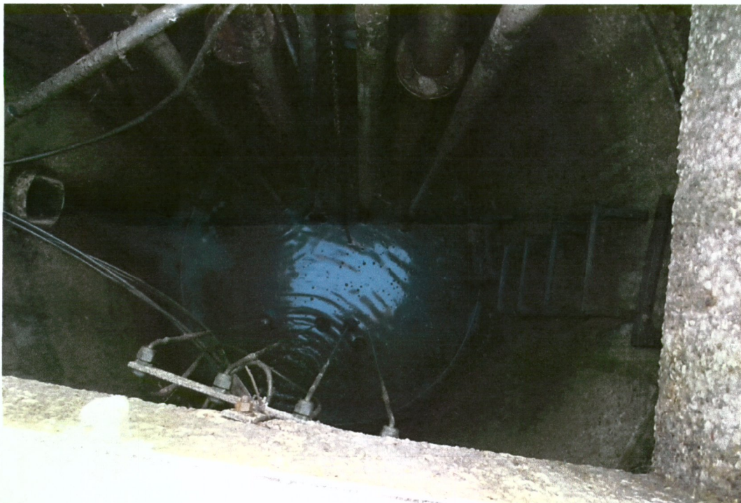
Pump Station #1 Interior
