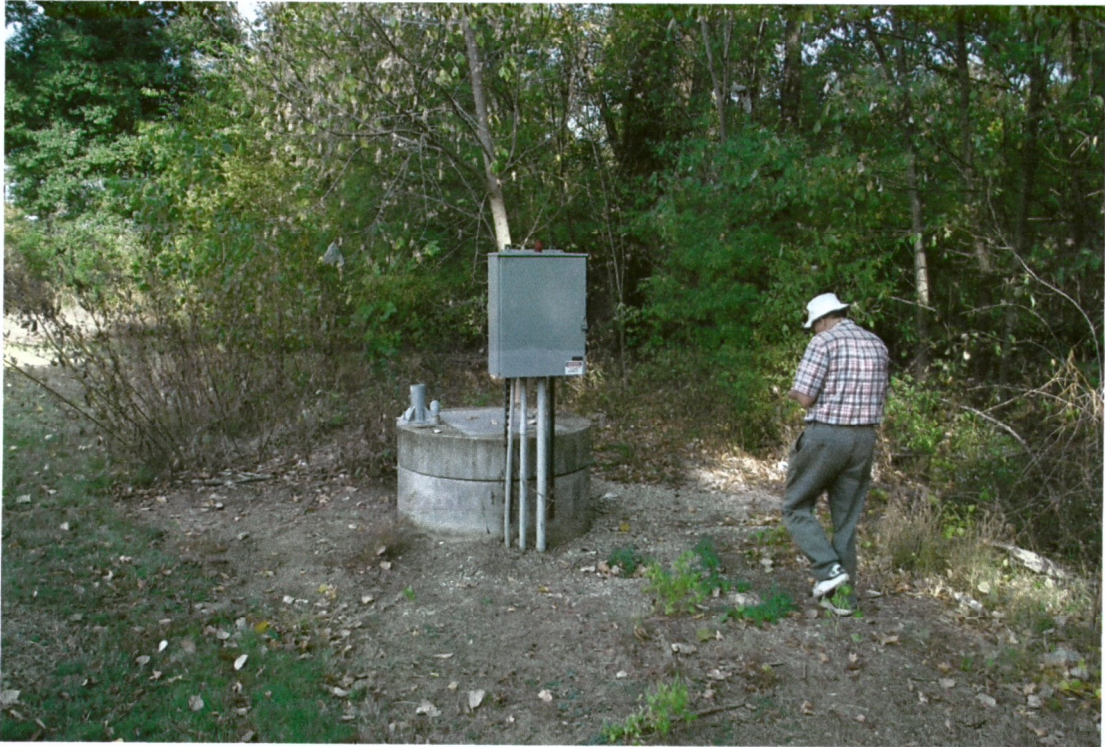
Pump Station #3 Exterior
