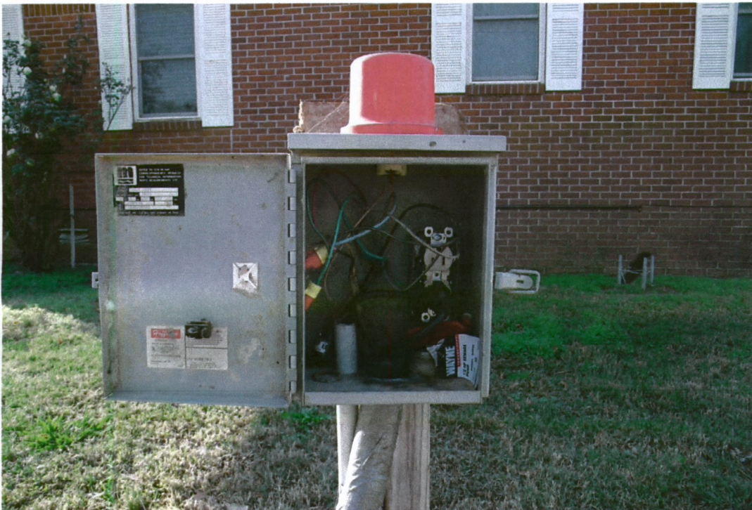
Grinder Pump at County Roads #712 & 716 Control Box (note emergency light still in need of repair)
