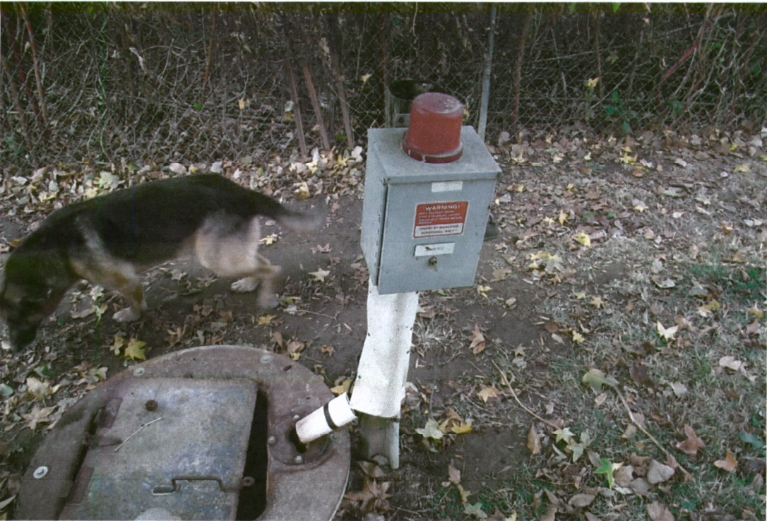
Grinder Pump on CR #712 (Lid still in need of repair and emergency light needs repair).
