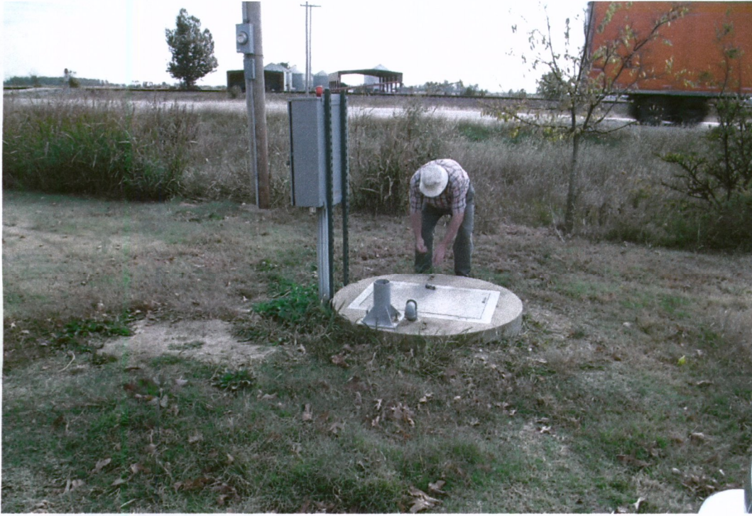
Pump Station #5 exterior
