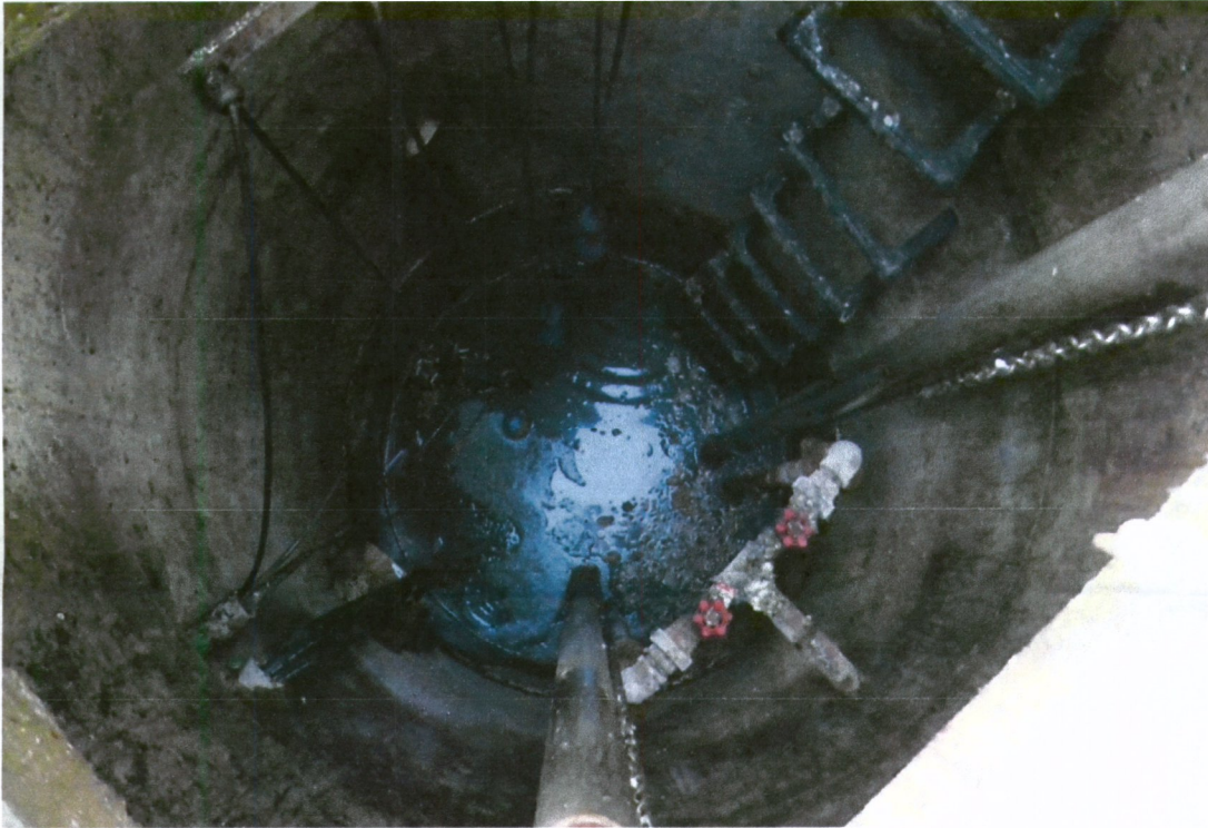
Pump Station #2 Interior
