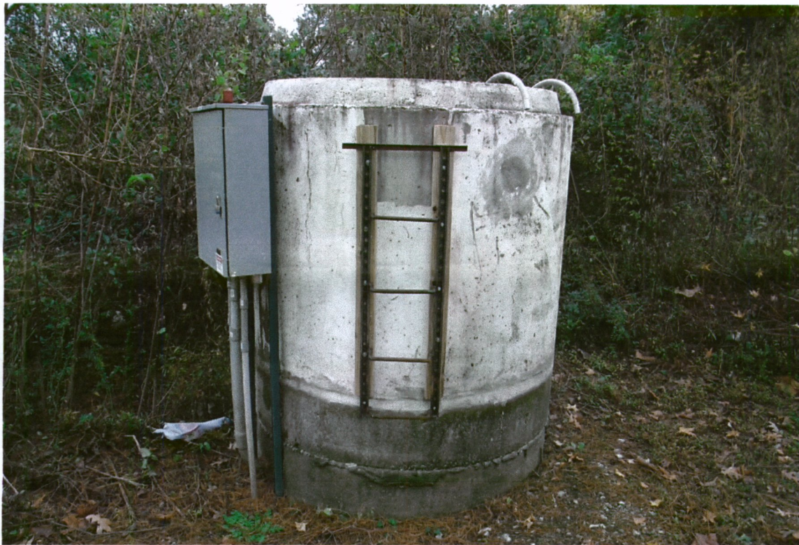
Pump Station #4 (note the permanent ladder).
