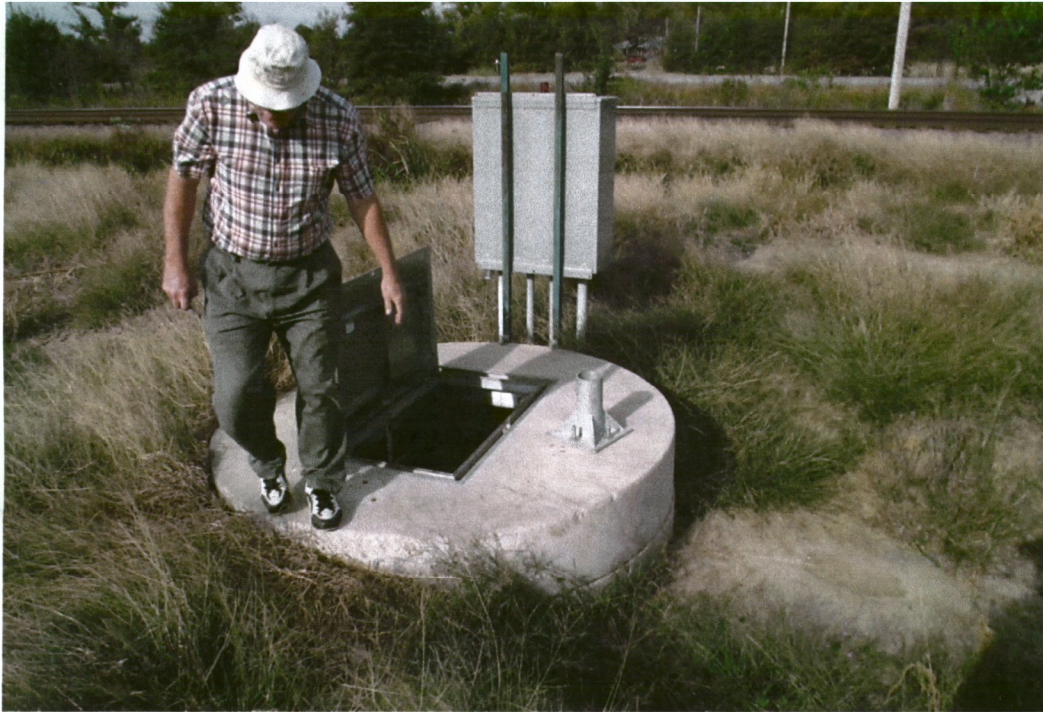
Pump Station #6 exterior
