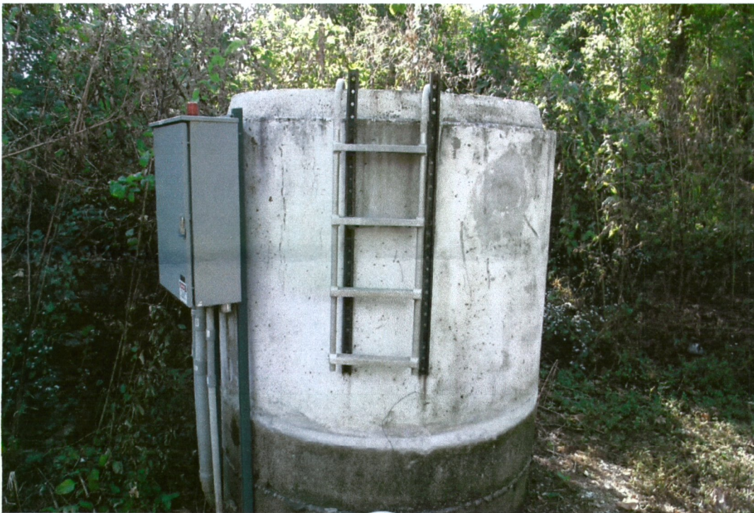
Pump Station #4 (note ladder, we are working on a more permanent solution)
