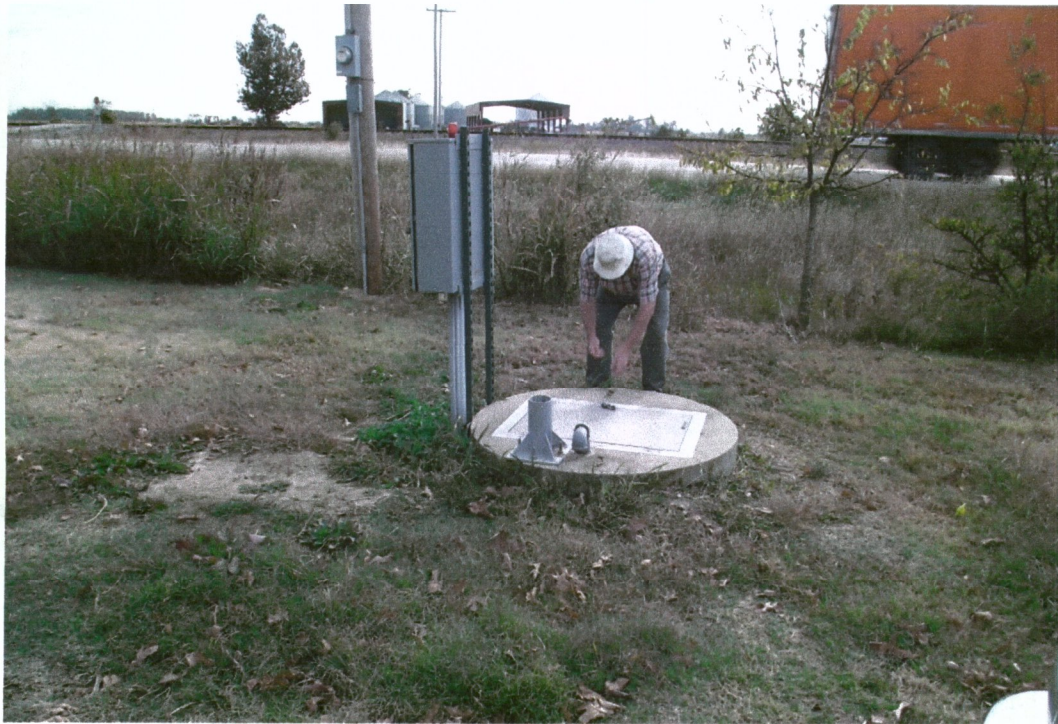
Pump Station #5 exterior
