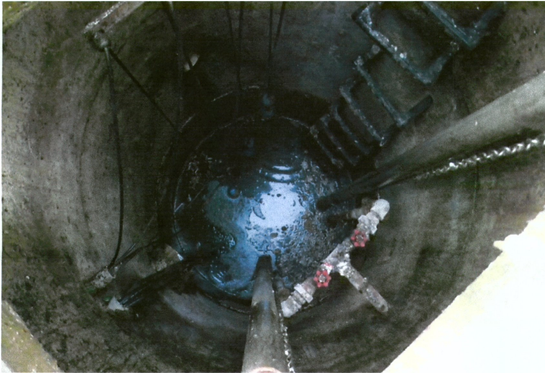
Pump Station #3 Interior (note excess grease removal)
