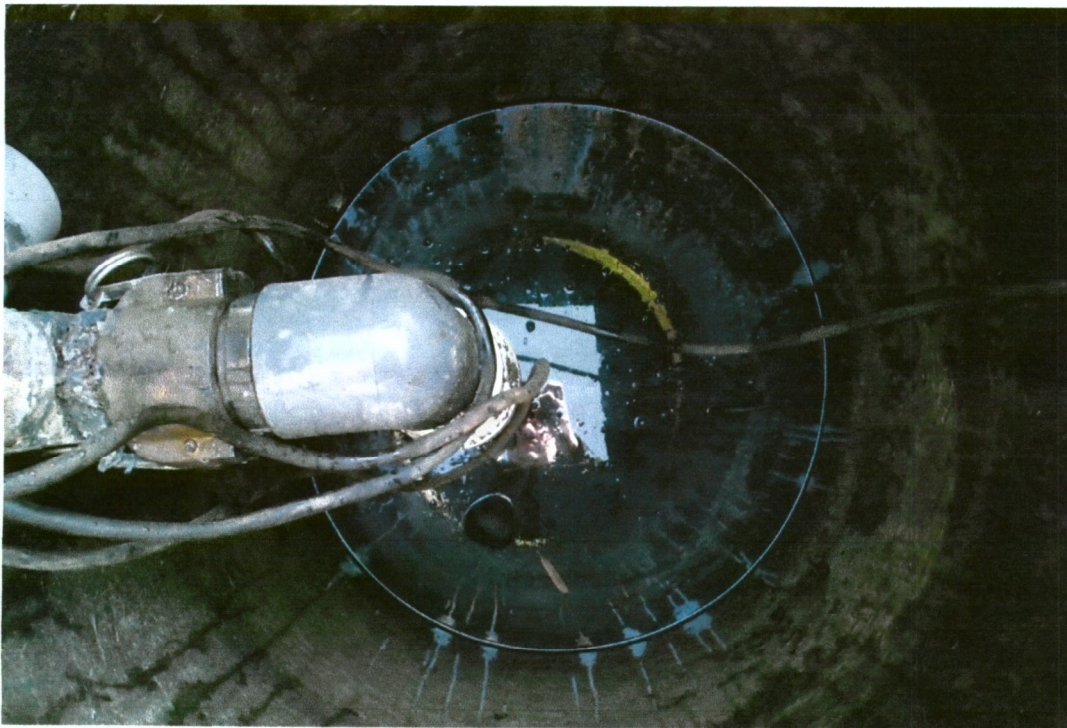
Grinder Pump at County Roads #712 & #716 (note water level down due to installation of new pump)
