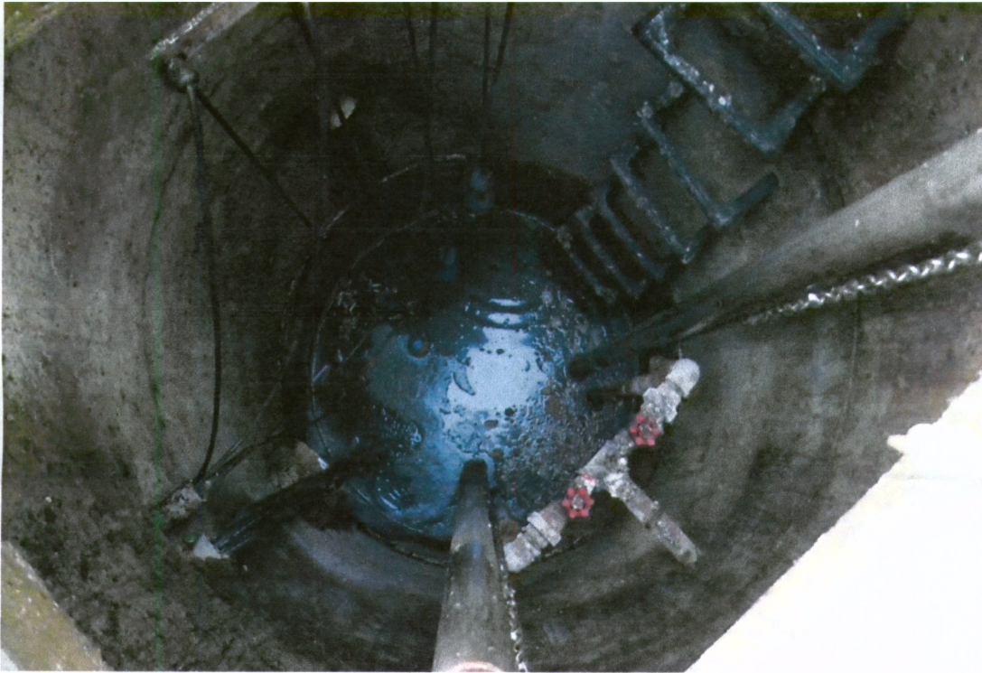
Pump Station #3 Interior (note excess grease removal)
