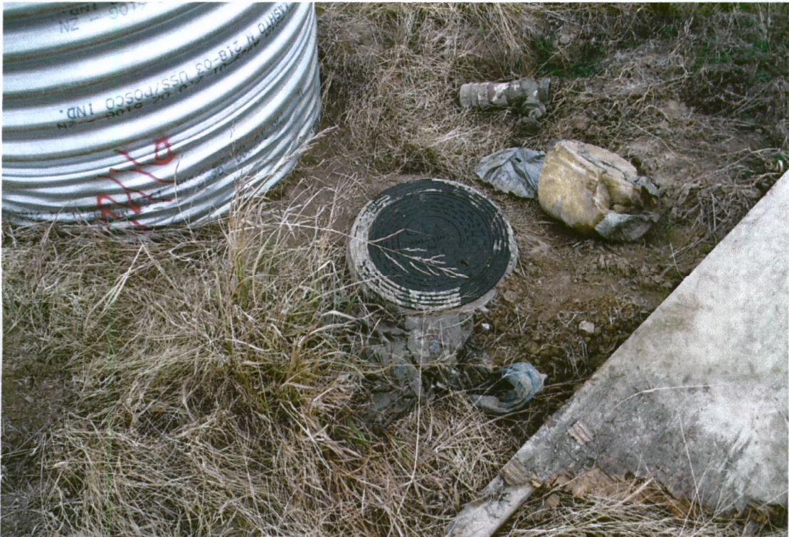
Pump Station #6 (note the new lid installed to replace the plywood cover.)
