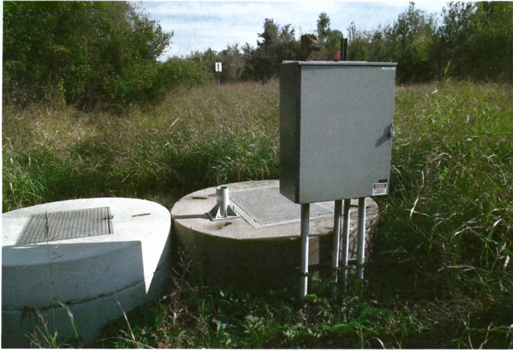
Pump Station #1 Exterior
