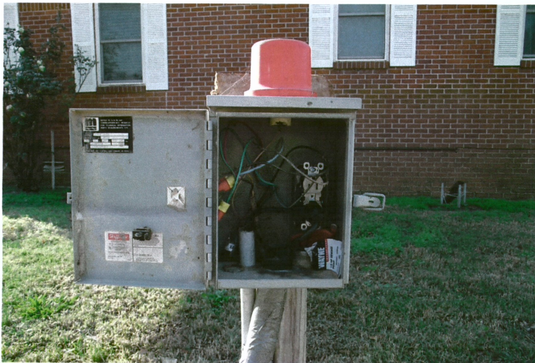
Grinder Pump at County Roads #712 & 716 Control Box
