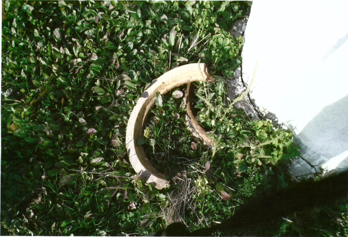
Old grout ring removed from manhole at pump station #2
