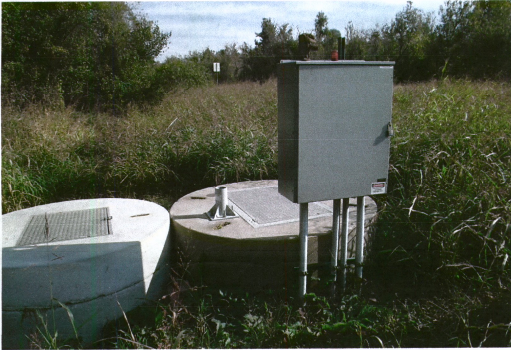
Pump Station #1 Exterior
