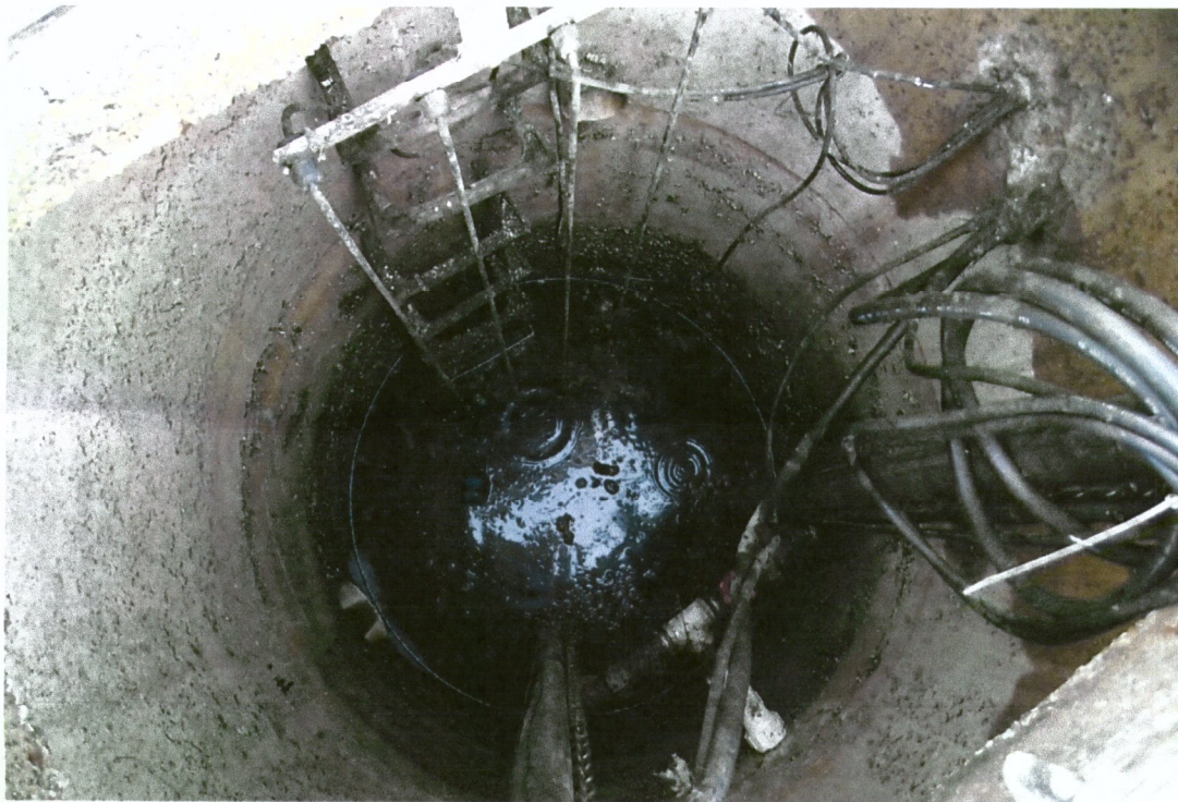
Pump Station #5 Interior
