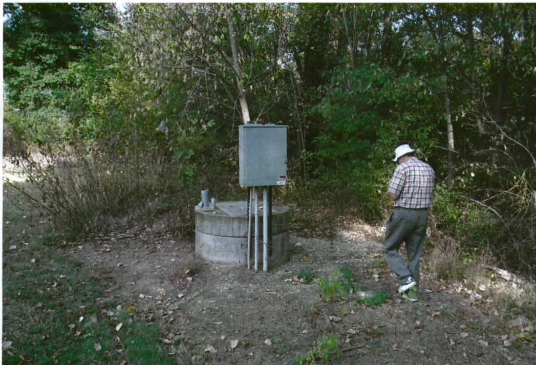
Pump Station #3 Exterior
