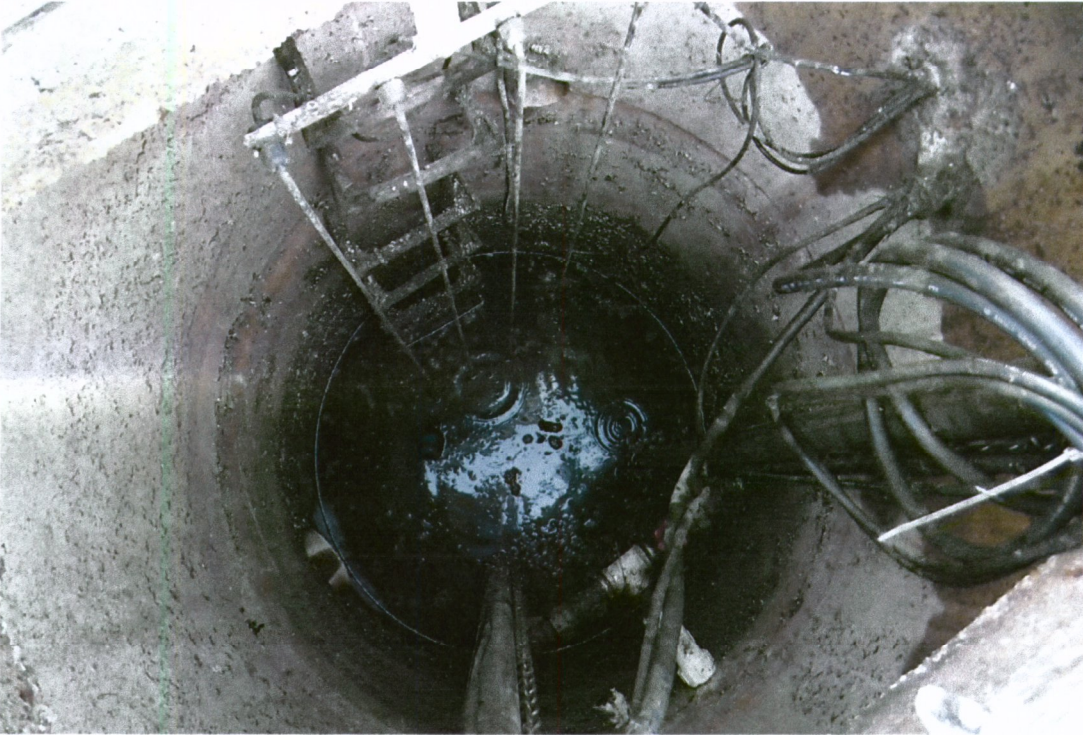
Pump Station #5 Interior
