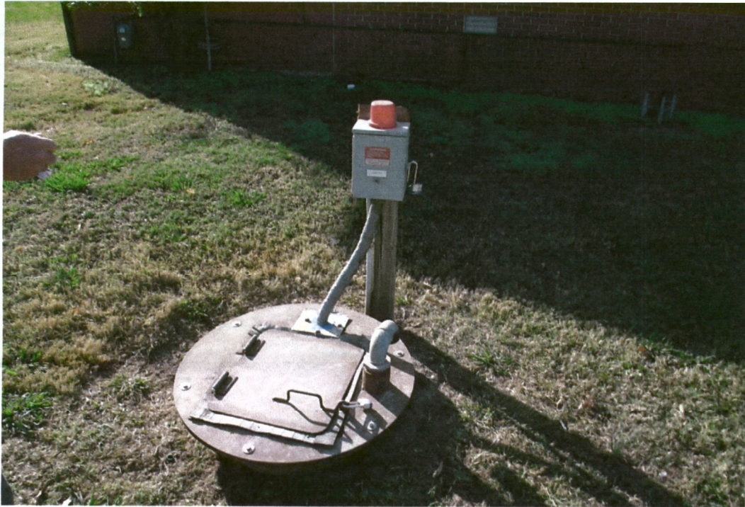
Grinder Pump at County Roads #712 and #716(note reconfiguration of post and installation of new lock on the control panel)
