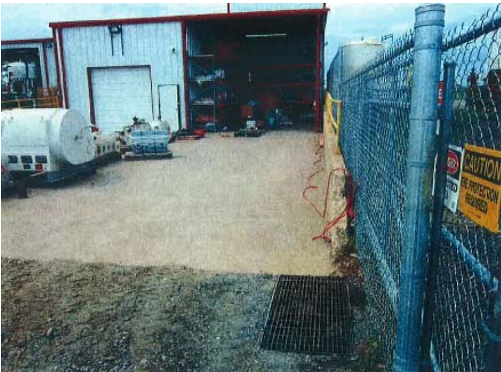
Photo 4: Catch basin with 4-inch diameter pipe at the end of the concrete driveway for the Maintenance Shop Building.
