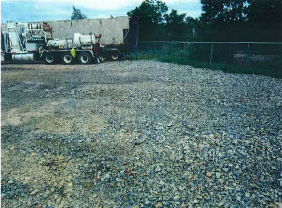
Photo 1: View of remediation conducted for oil-stained gravel in Southern portion of Facility. Backfilled after excavated (Note: ADEQ, Item No. 13).
