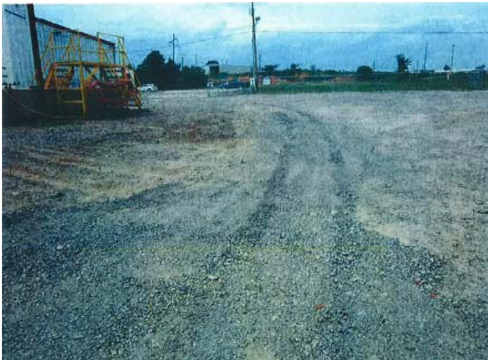
Photo 6: Fill and grade in center of the Property to influence proper drainage.
