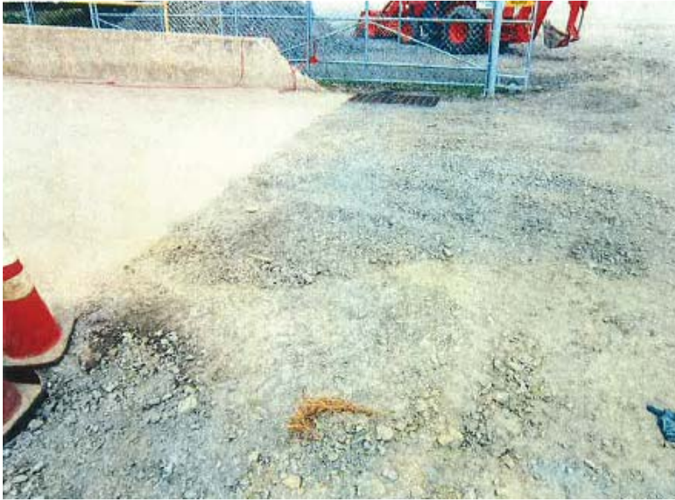
Photo 5: Fill and grading to control storm water flow at the end of the driveway for the Maintenance Shop Building.
