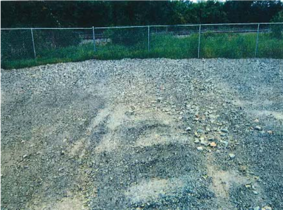
Photo 2: View of final grade and backfill for excavated oil-stained gravel in Southern portion of Facility (Note: ADEQ Item No. 13).
