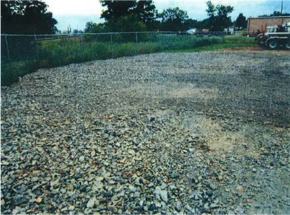
Photo 3: View looking west for remediation conducted in Southern portion of the Facility.
