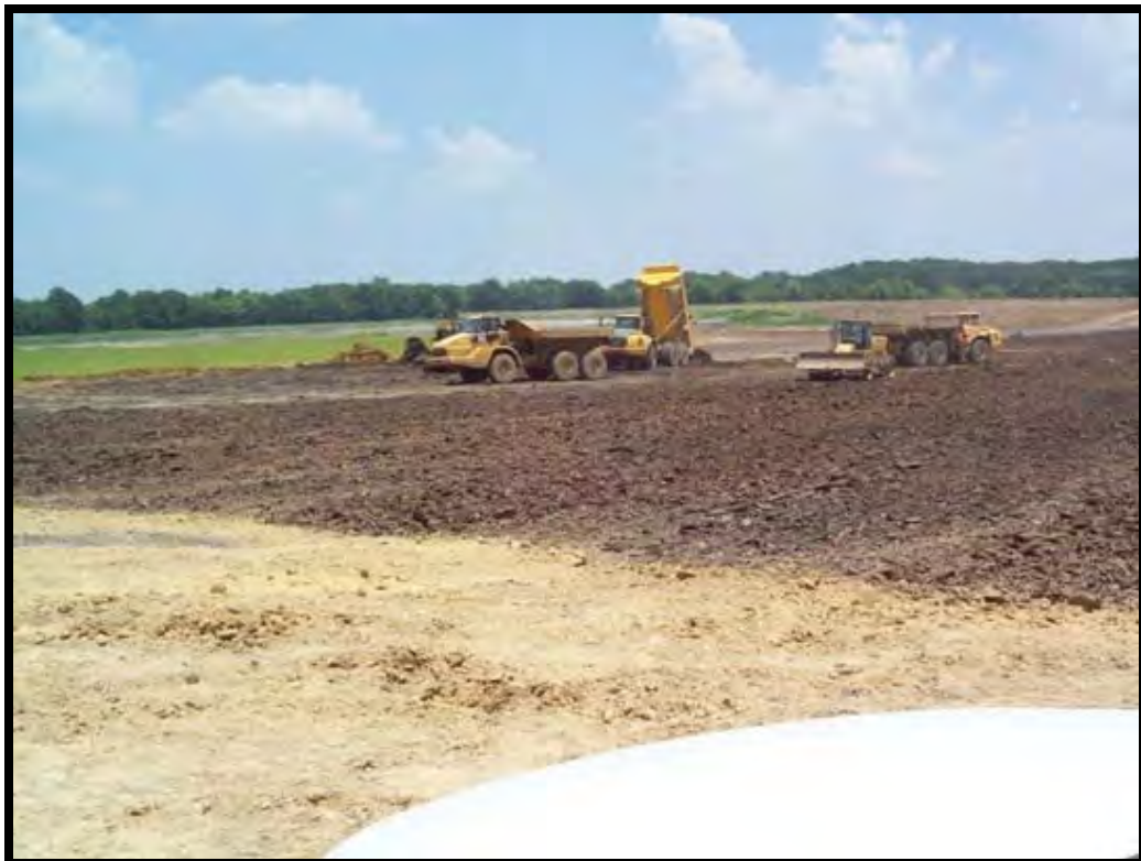
Looking east at installation of subgrade
