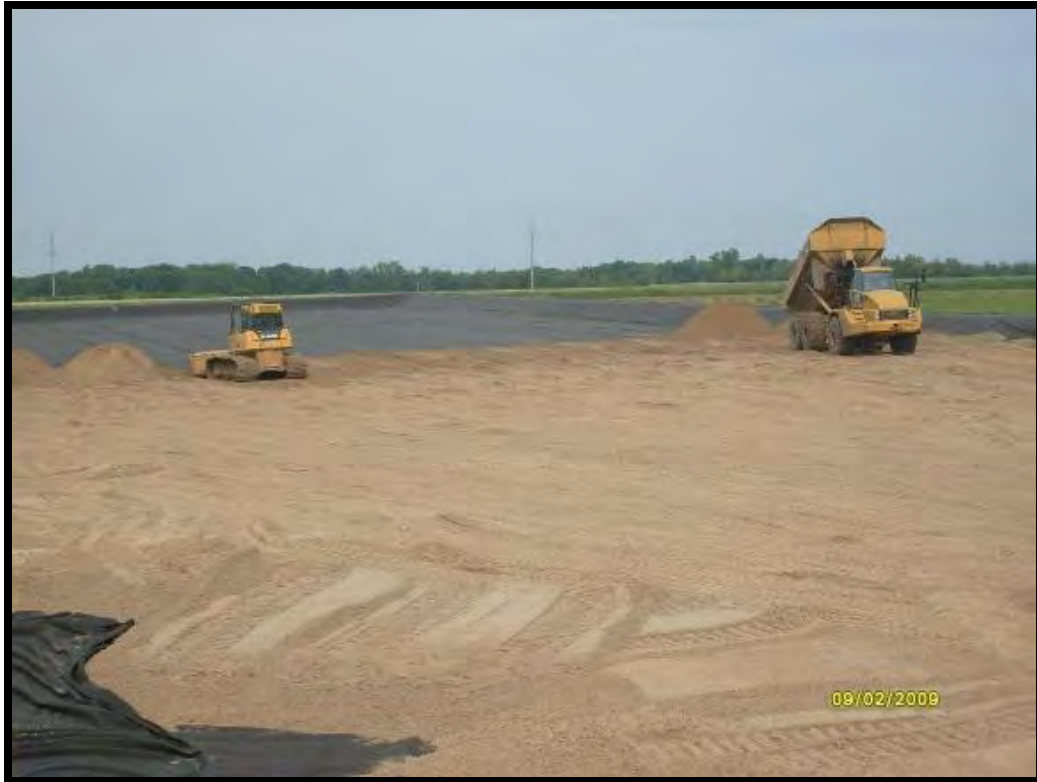
Looking west at installation of 18-inch thick sand protective cover layer
