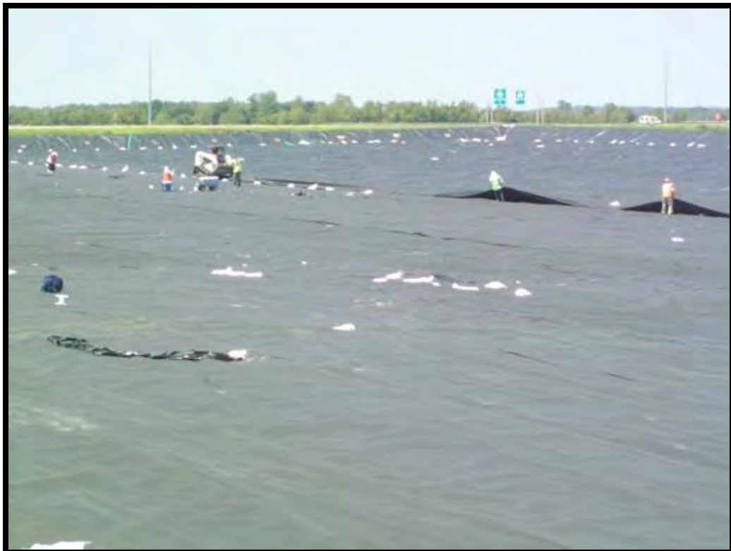
Deployment of 8 ounce double sided geocomposite drainage layer
