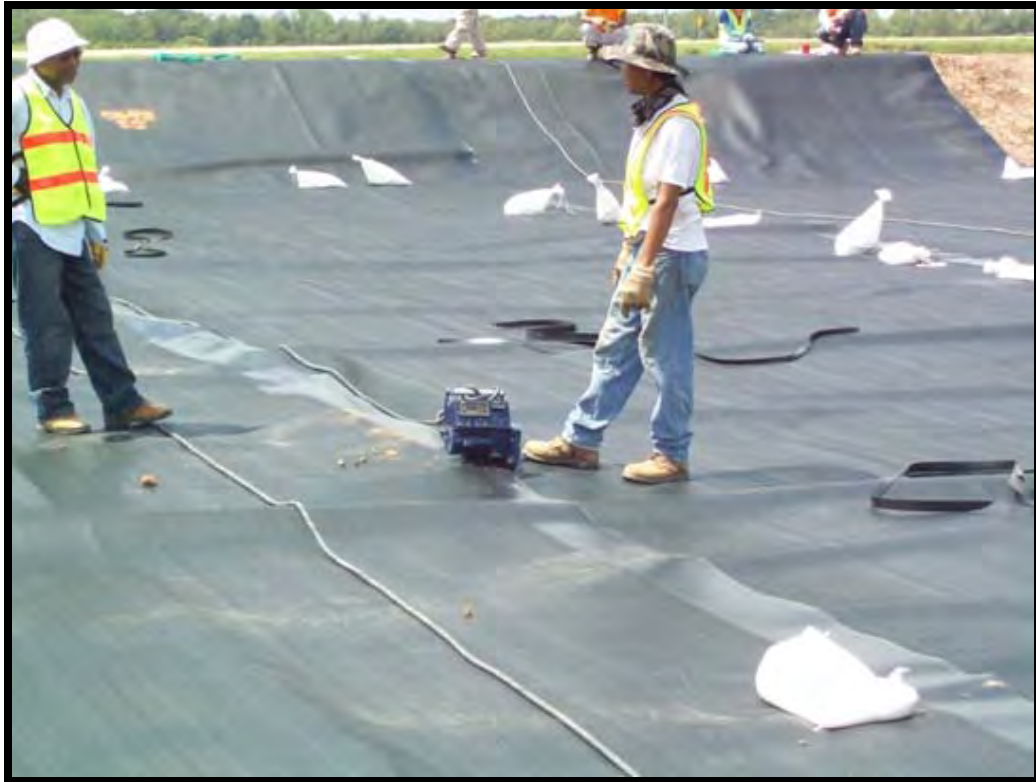
Continued installation of 60-mil HDPE geomembrane liner
