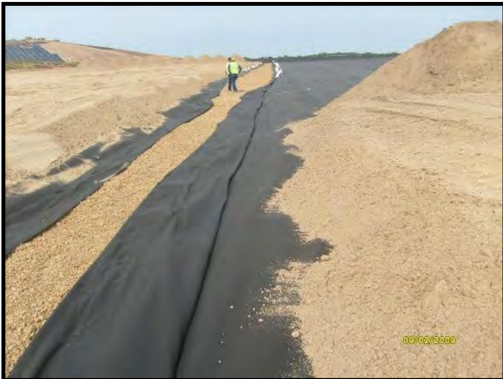
Looking west at installed leachate collection trench
