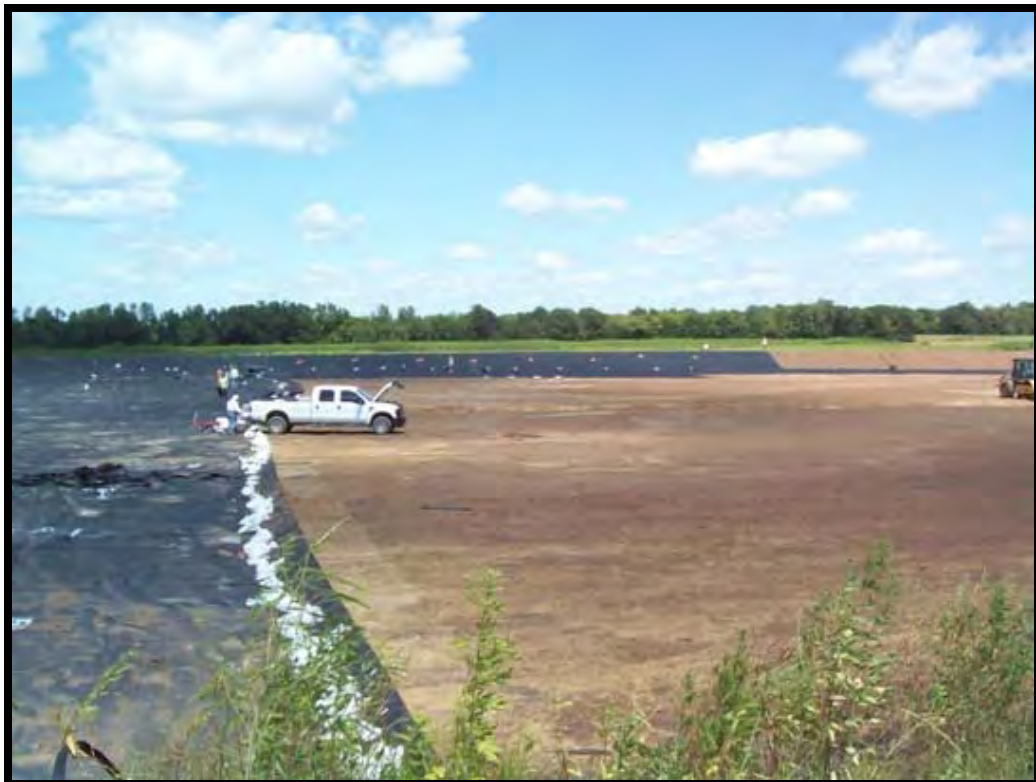
Looking north at installation of 60-mil HDPE geomembrane liner
