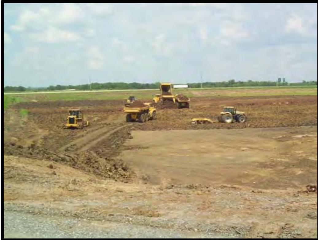
Looking west at installation of subgrade
