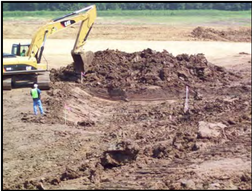
Excavation of leachate collection sump
