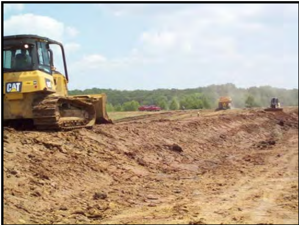
Construction of north overbuild berm
