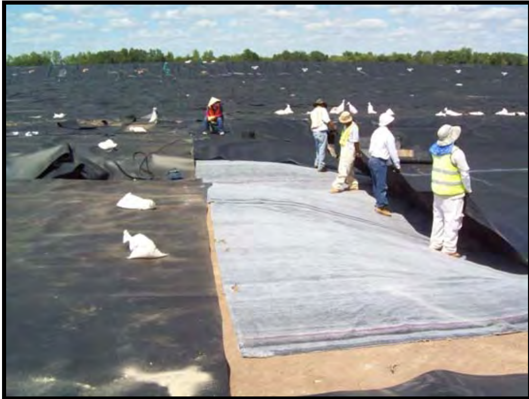
Installation of geosynthetic clay liner and double geomembrane liner in leachate sump
