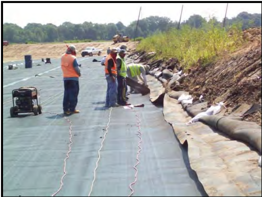
Completing tie-in to existing Cell 1 liner system
