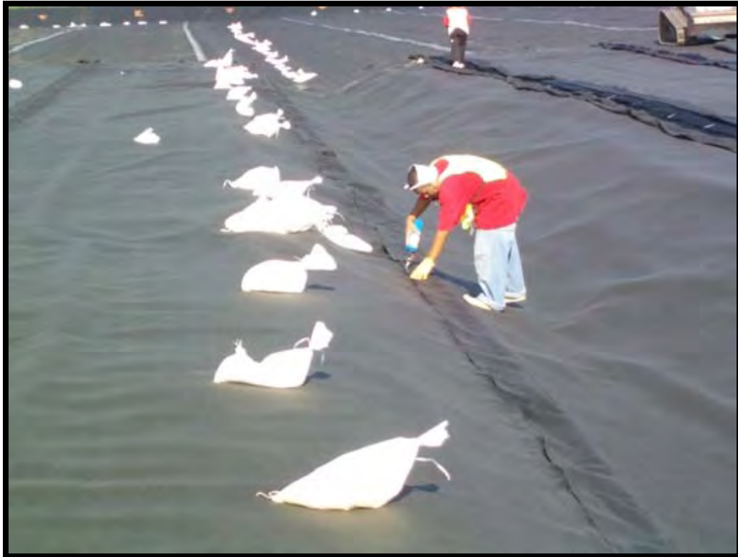
Completing installation of 8 ounce double sided geocomposite drainage layer
