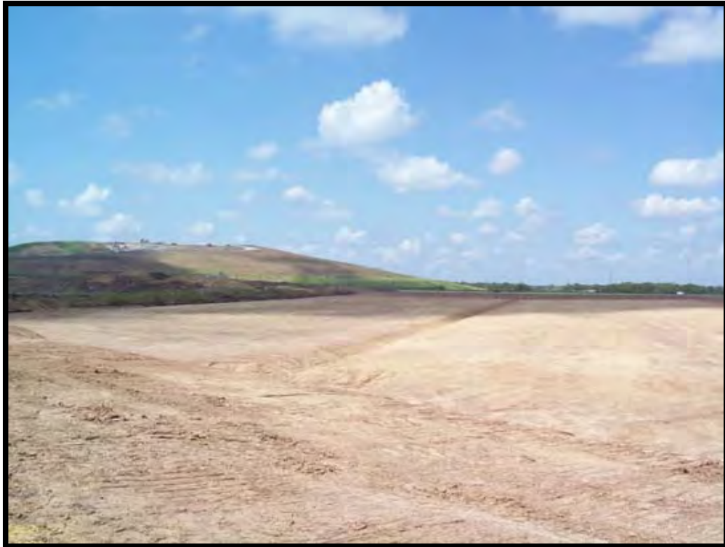
Looking west at completed compacted clay liner system
