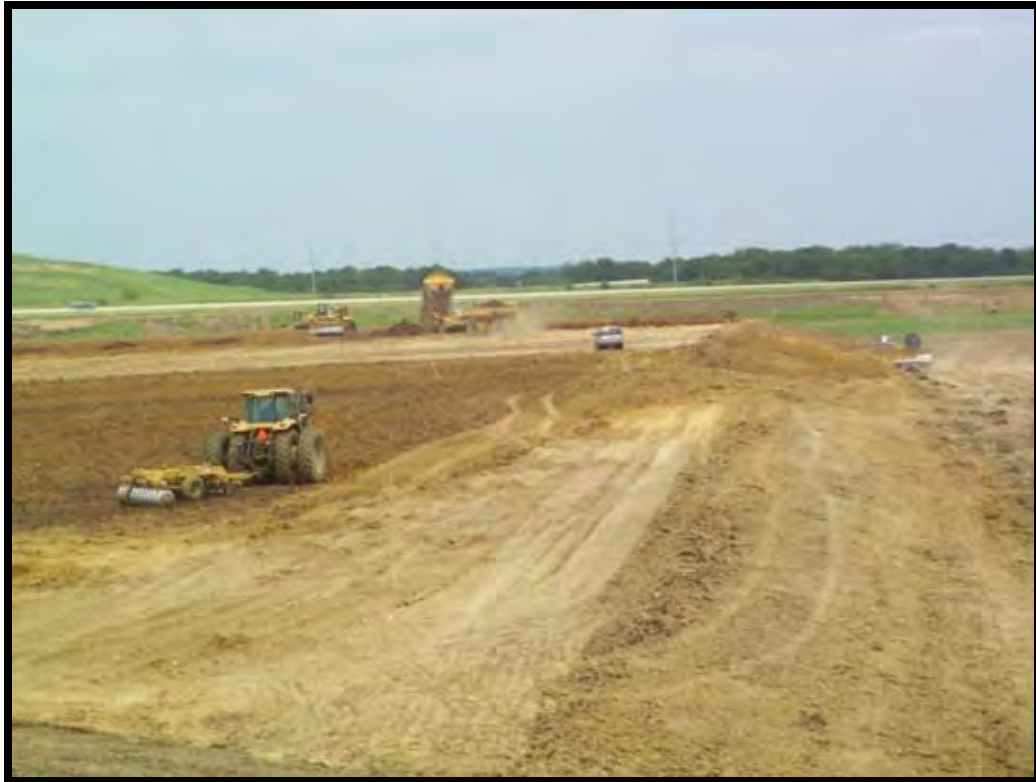
Looking west at installation of compacted clay liner system
