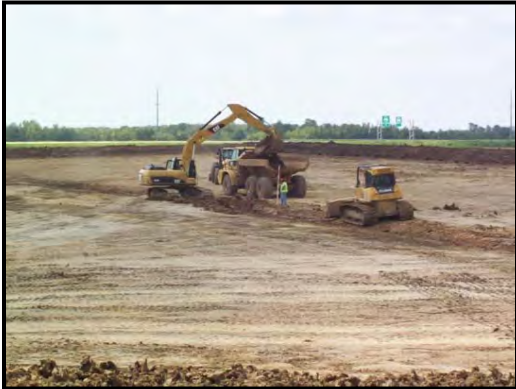
Construction of leachate collection trench
