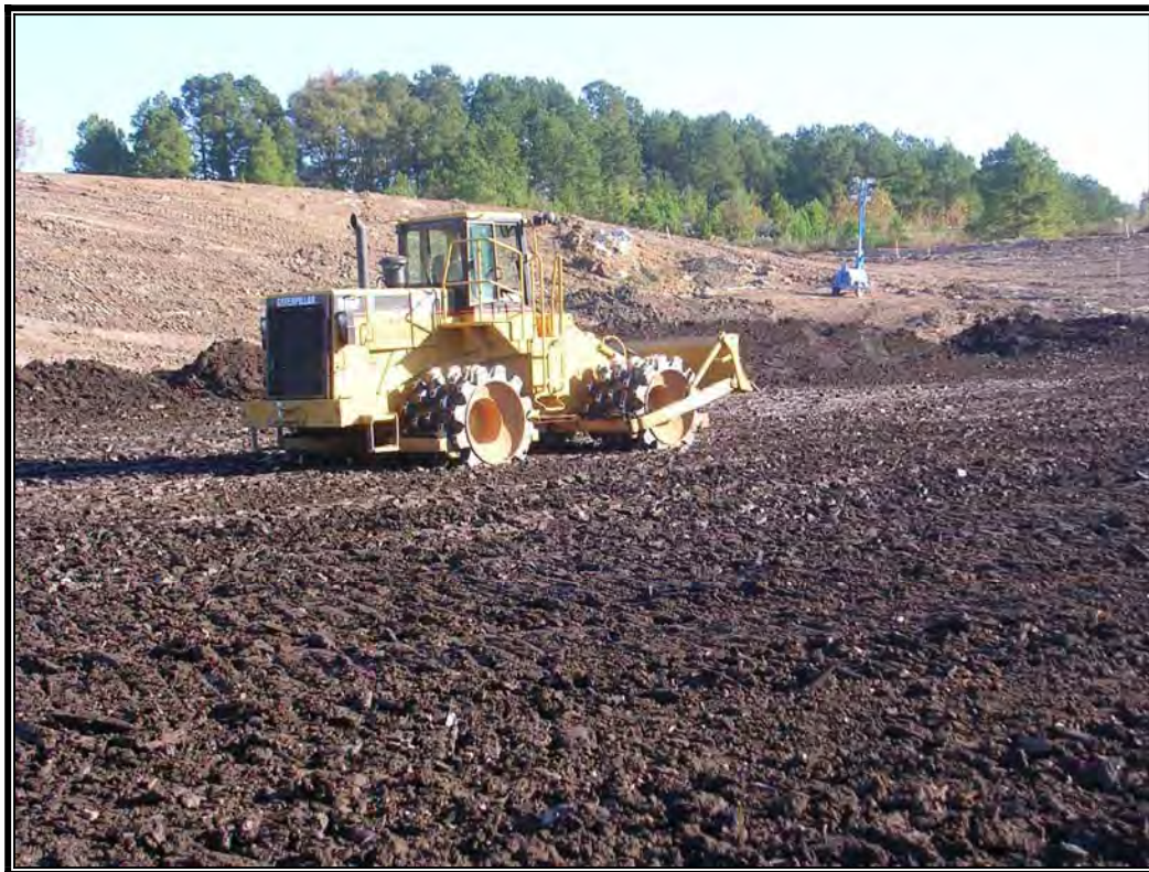
Installation of compacted clay liner
