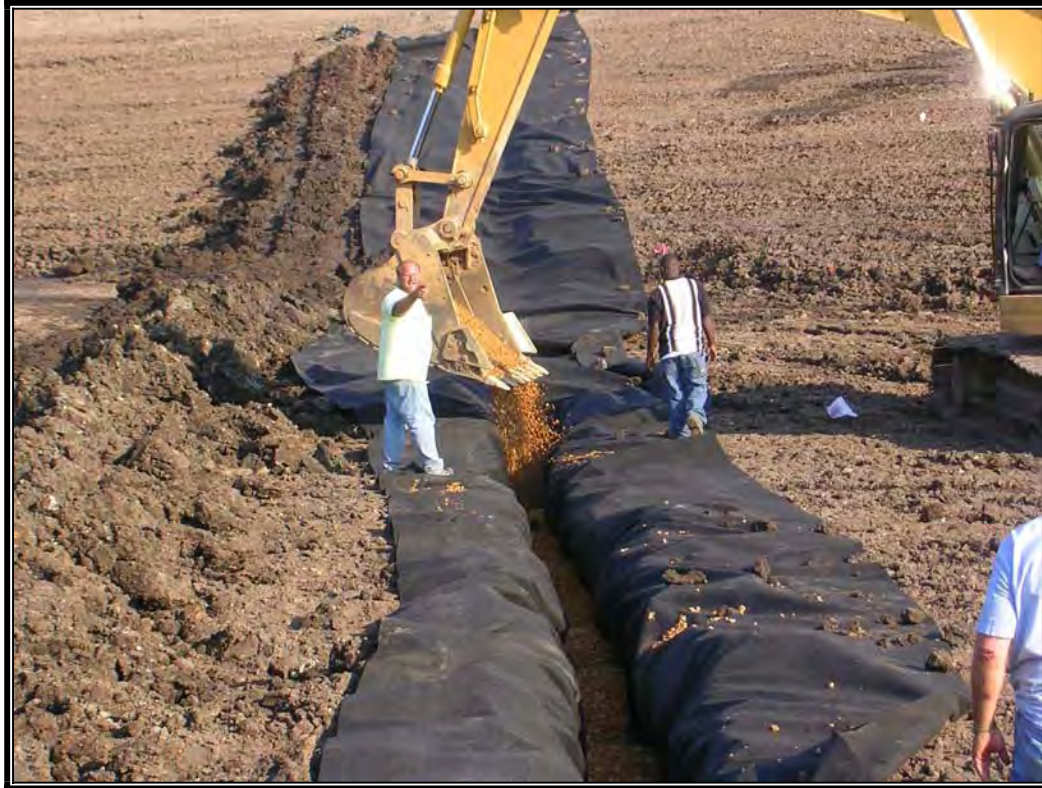
Installation of geotextile and gravel in under-drain system
