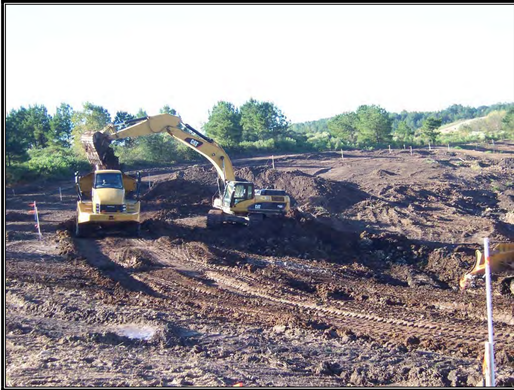
Looking southeast at excavation of Phase II
