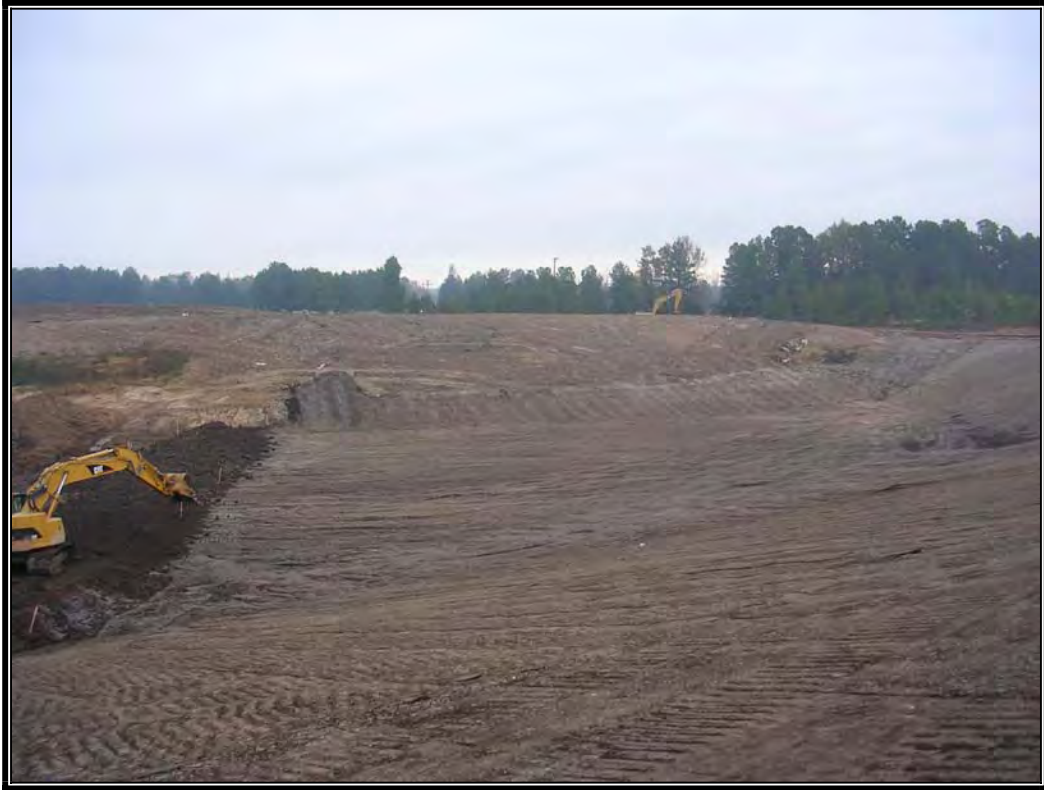
Looking north, construction of west perimeter cell berm
