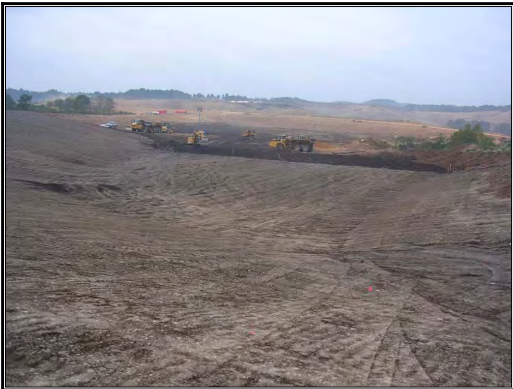
Looking west at top of clay liner
