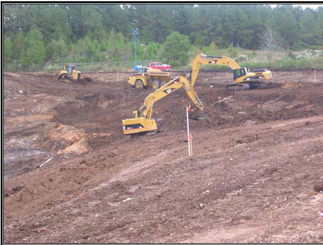
Looking northeast at continued excavation of Phase II
