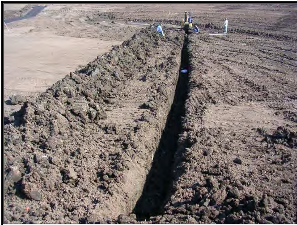
Excavation of under-drain system trench
