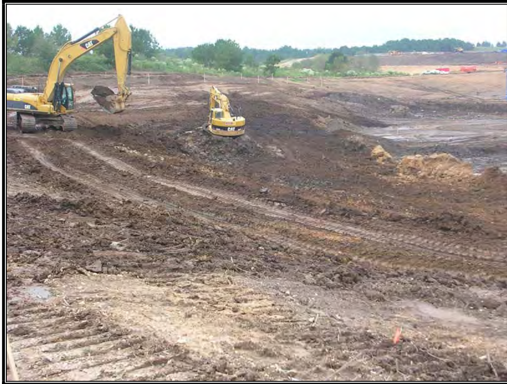
Excavation and installation of subgrade layer
