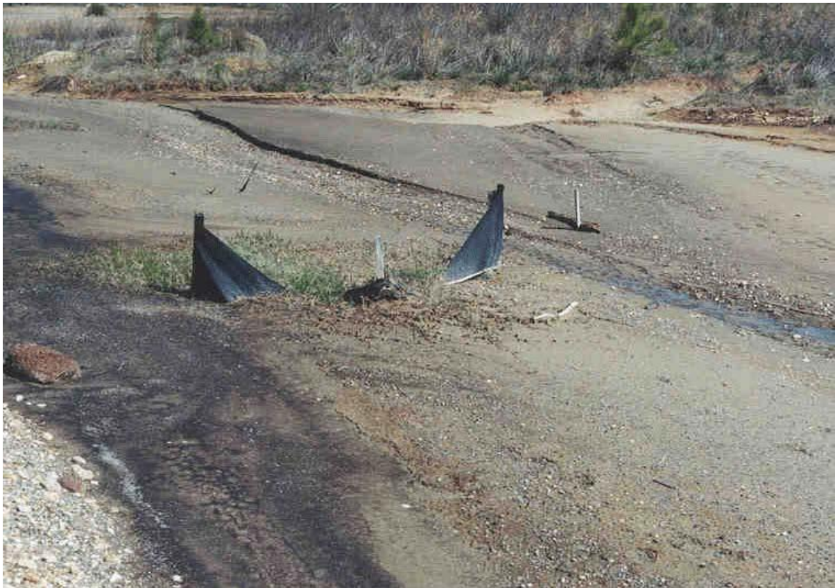
Figure 4-2: Ineffective Silt Fence
