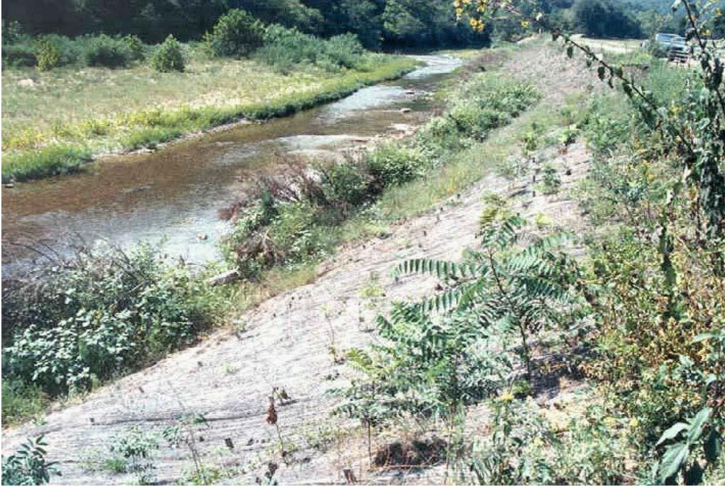
Figure 6-3: Geotextile used for stream bank stabilization
