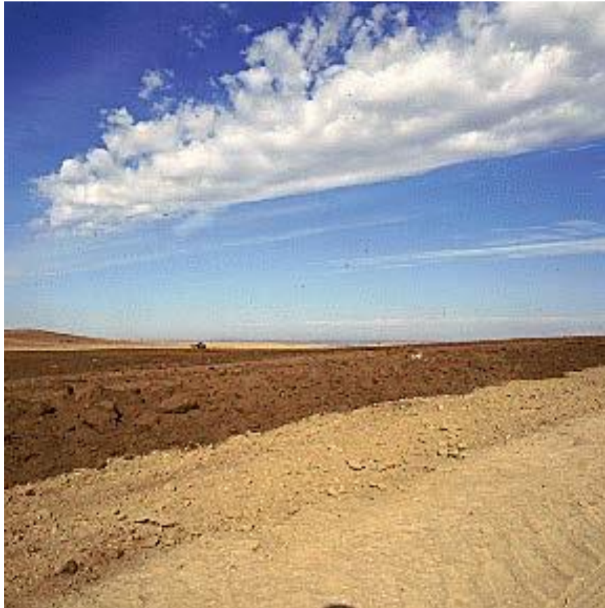
Figure 5-2: Topsoil replacement (from OSM website photo gallery)
