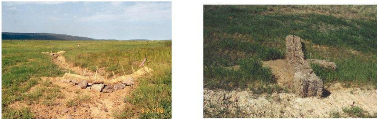
Figure 4-4: Hay Bale erosion control structures
