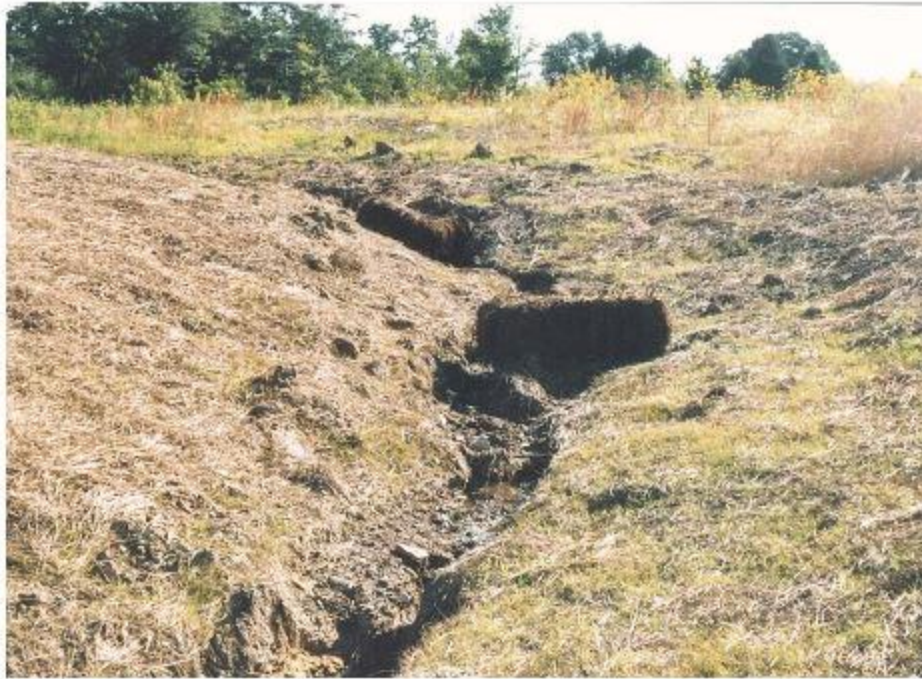
Figure 4-5: Improper installation of hay bales as erosion control structure
