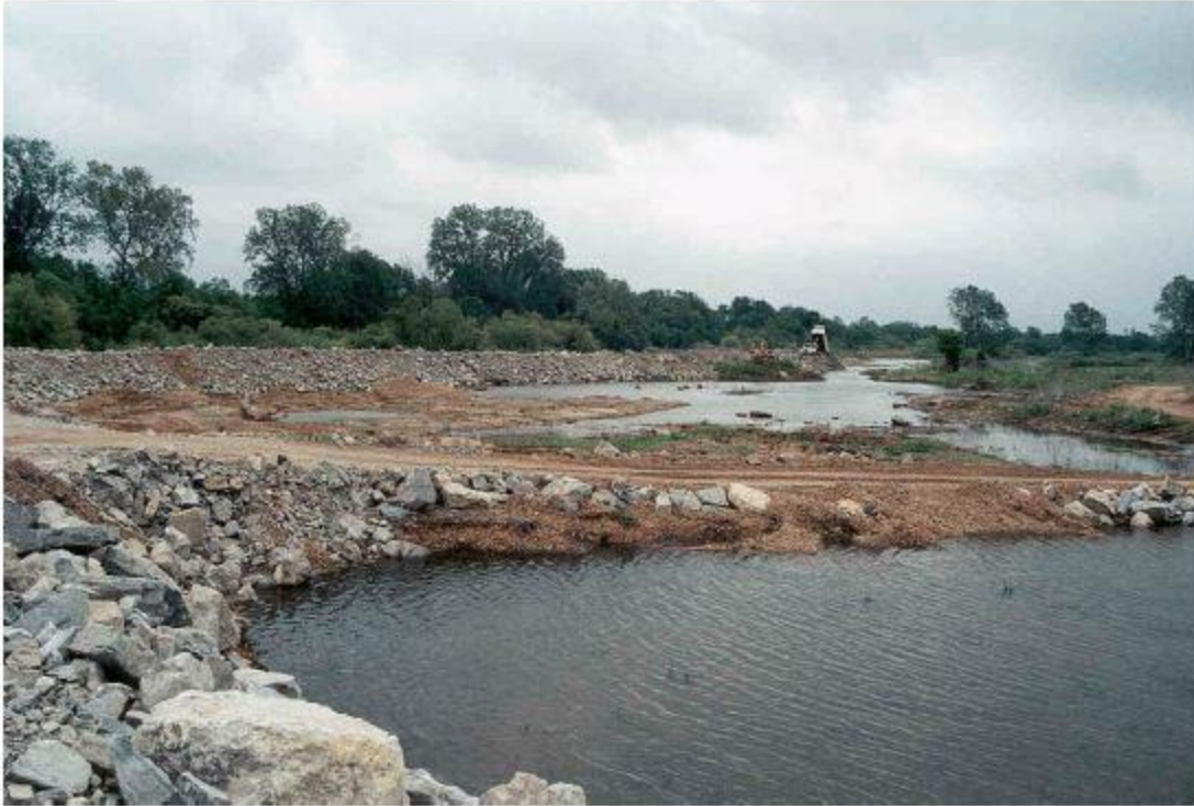
Figure 4-10: Riprap berm
