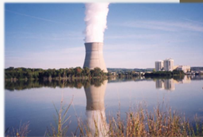
Industrial Water Supply
