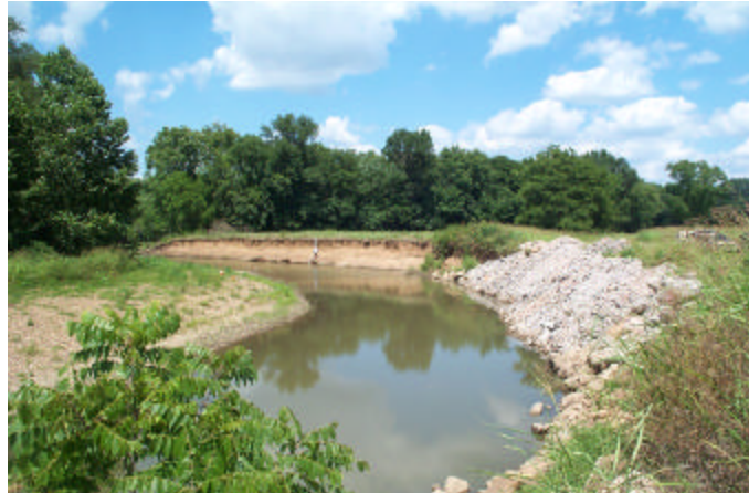
Figure 4-12 Eroding bank at Reach #7 and the use of construction debris for bank stabilization
