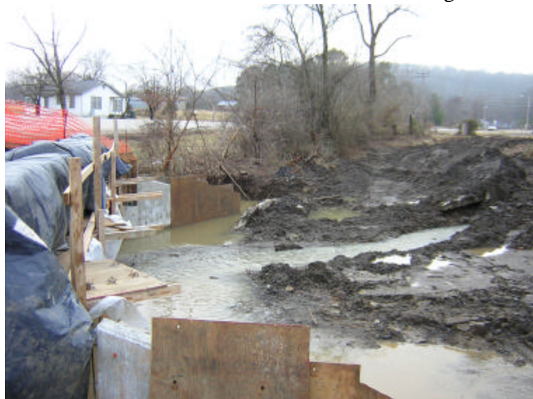
Figure 5-26 Construction site without proper BMPs in place to reduce sediment runoff.
