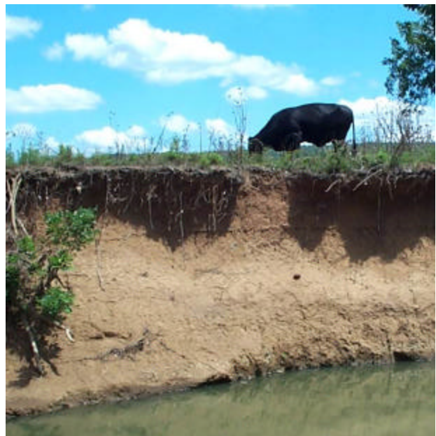
Figure 5-28 Numerous cattle operations exist in the WFWR watershed
