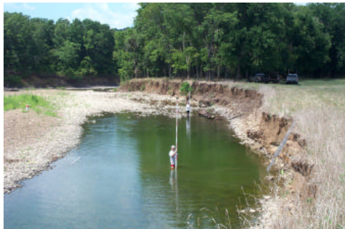
Figure 4-10 Lateral erosion of channel at Reach #5. Surveyors are standing where the toe of the streambank was located the previous year.
