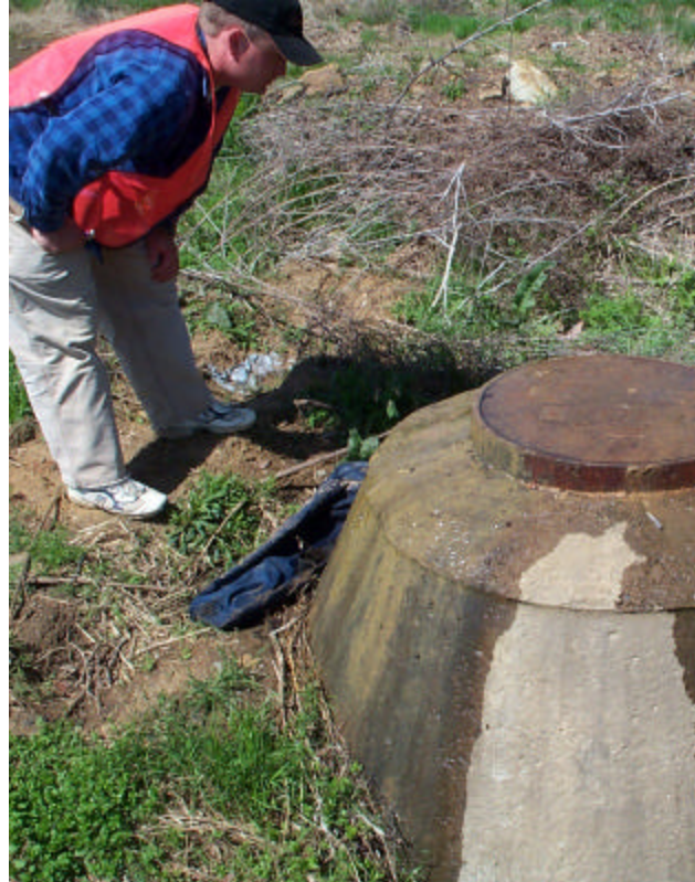
Figure 5-32 Leaking wastewater infrastructure can contribute nutrients to the watershed
