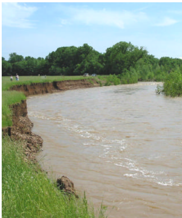
Figure 5-1 Eroding streambank at inventoried reach WF4
