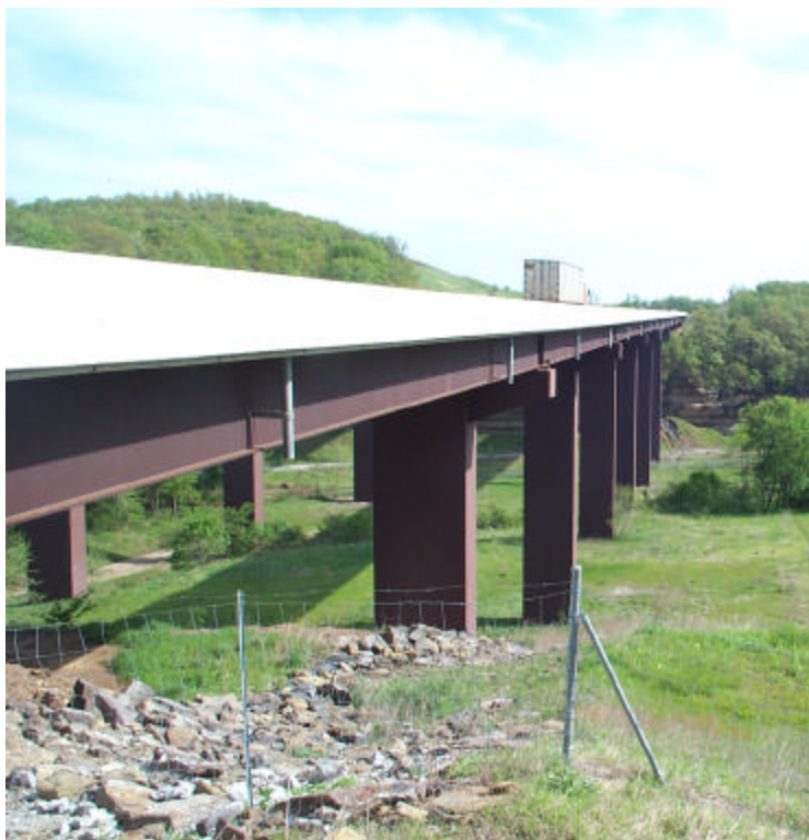
Figure 5-19 Winn Creek Bridge south of the town of West Fork
