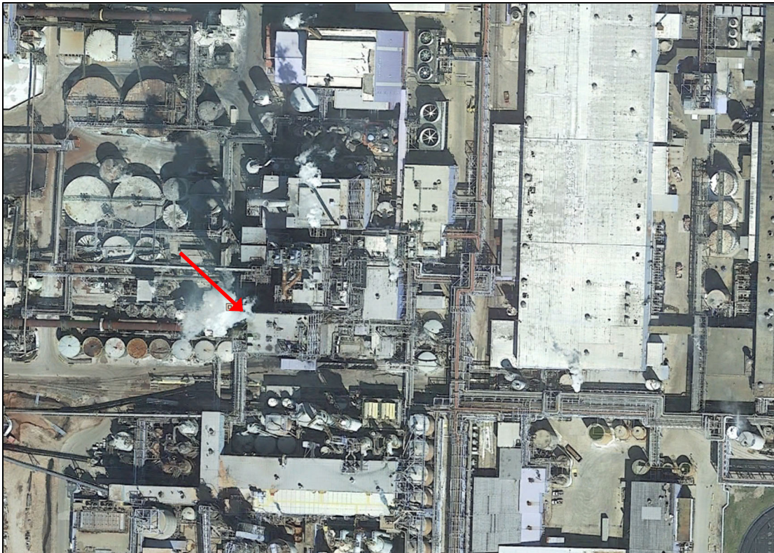
Figure 3-2. Aerial Showing No. 2 Power Boiler and Surrounding Equipment
