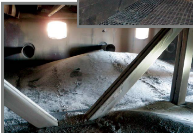
Ash deposits are a common problem in SCR systems, which can be alleviated through the application of fluid dynamics and utilizing baffling and screening hardware.
