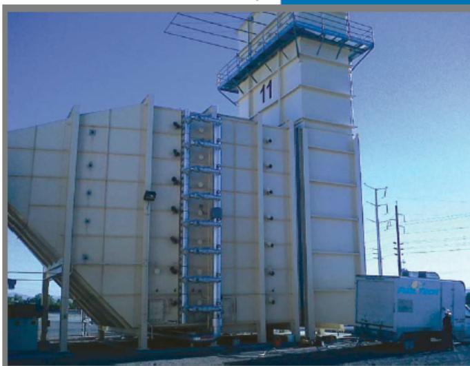
Selective Catalyst Reduction systems help prevent the release of nitrogen oxides from a variety of power and industrial processes. A Simple Cycle Combustion Turbine SCR is shown here.
