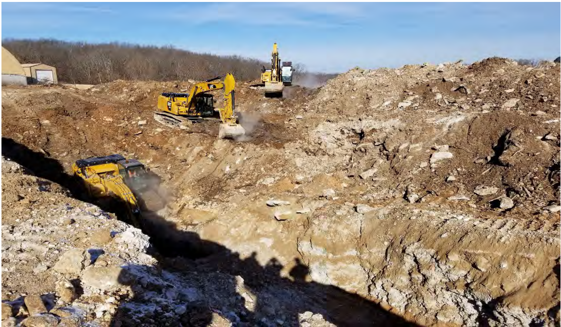
Photo 2: Trench excavation procedures, showing benched excavation. To achieve excavation to depths >40 feet bgs, the trench was widened. One trackhoe excavated material to mid-depth. A second trackhoe lifted material to near ground surface. A third trackhole manipulated material into the debris stockpile. Note stumps and concrete in stockpile.
