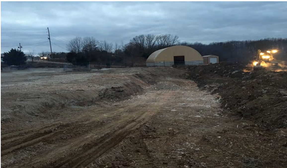
Photo 10: The trench and south bench area (view to west); fill and compaction activities occurring on north bench. Segregated soil from the debris pile was used to fill the north bench.
