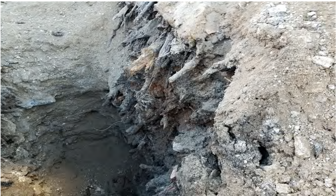
Photo 6: Close up of deep debris layer approximately 30-40 feet bgs (compacted soil, tree trunks, etc.)
