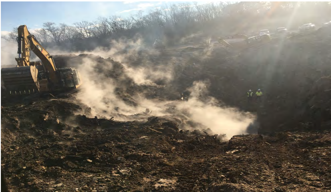
Photo 4: Smoke vent with steam approximately 25 feet bgs encountered on 27 January 2019. EnSafe personnel performing air monitoring of trench.
