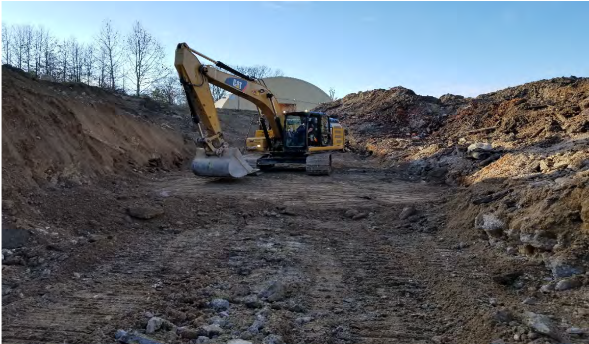
Photo 9: Filling trench to construct fire break (view to west). Clean fill material from on- and offsite was used to construct the subgrade fire break and to cover the south bench. The minimum cover over the waste was 5 feet; the minimum width of the trench was 5 feet.
