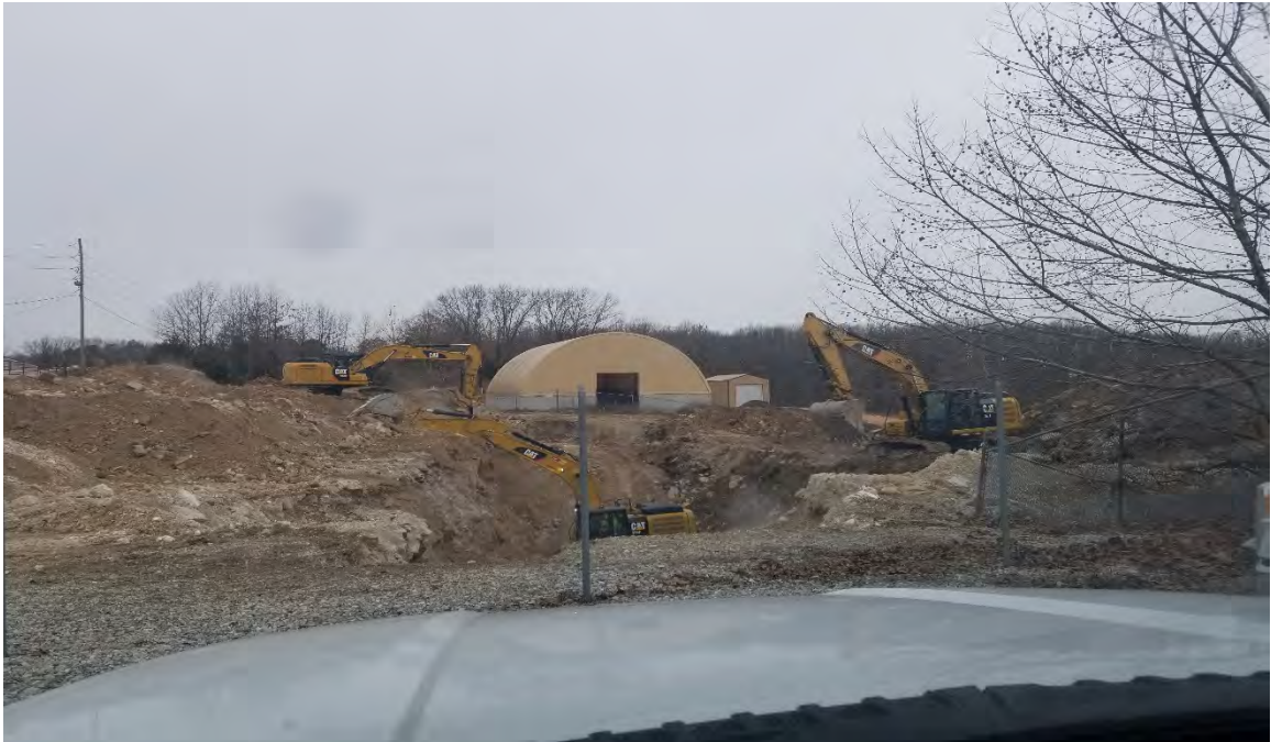
Photo 1: Trench excavation (view to west). Stockpile to south (left of photo) is segregated onsite “clean” soil from 0-15-foot bgs interval, and offsite clean fill. Stockpile to north (right of photo) is debris pile.
