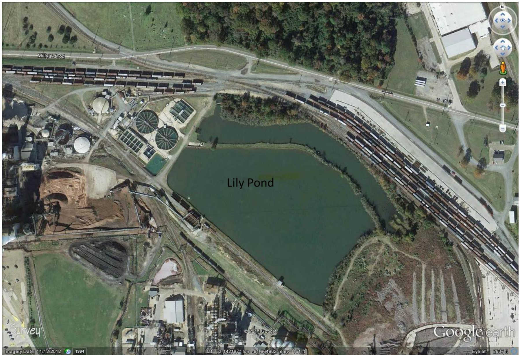
Figure 1. Google Earth image dated Nov 12, 2012 of overview of Lily Pond, which is used as process water for Georgia Pacific, LLC in Crossett, AR.
