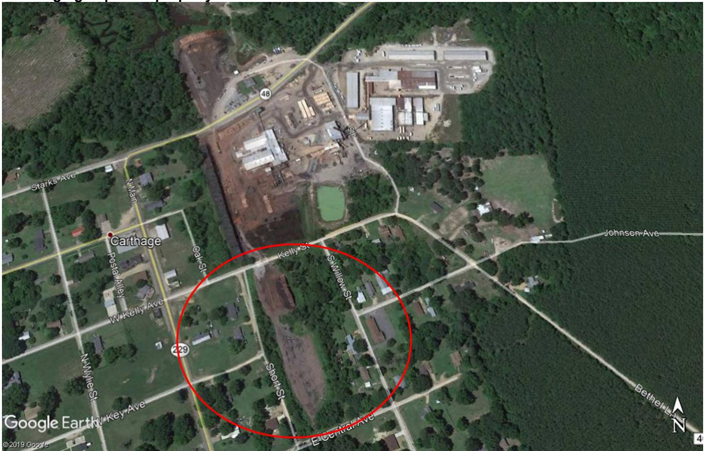
Figure 1. Overview of Idaho Timber of Carthage and the location of the wet-deck that was stated to be discharging to private property.
