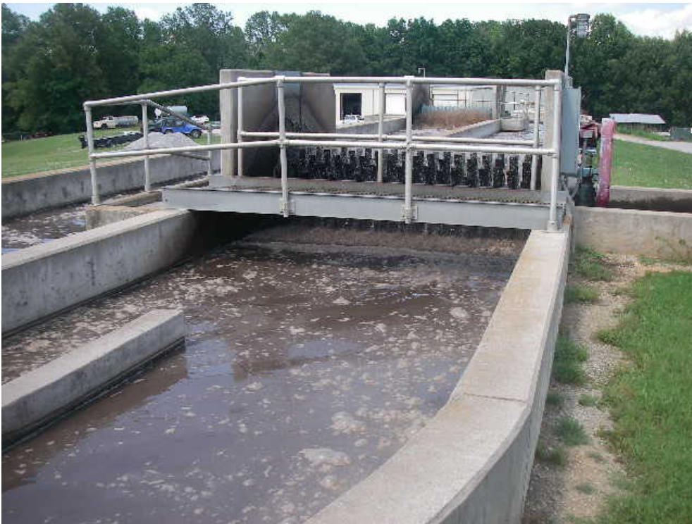
oxidation ditch:
