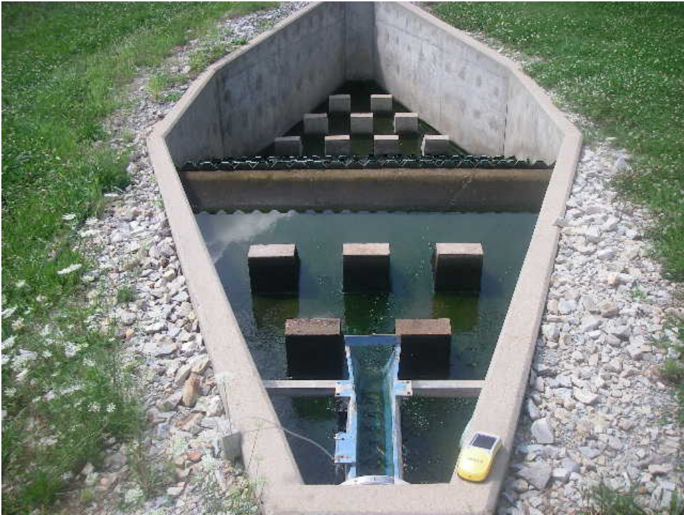
flow meter (foreground, post aeration in the background)
