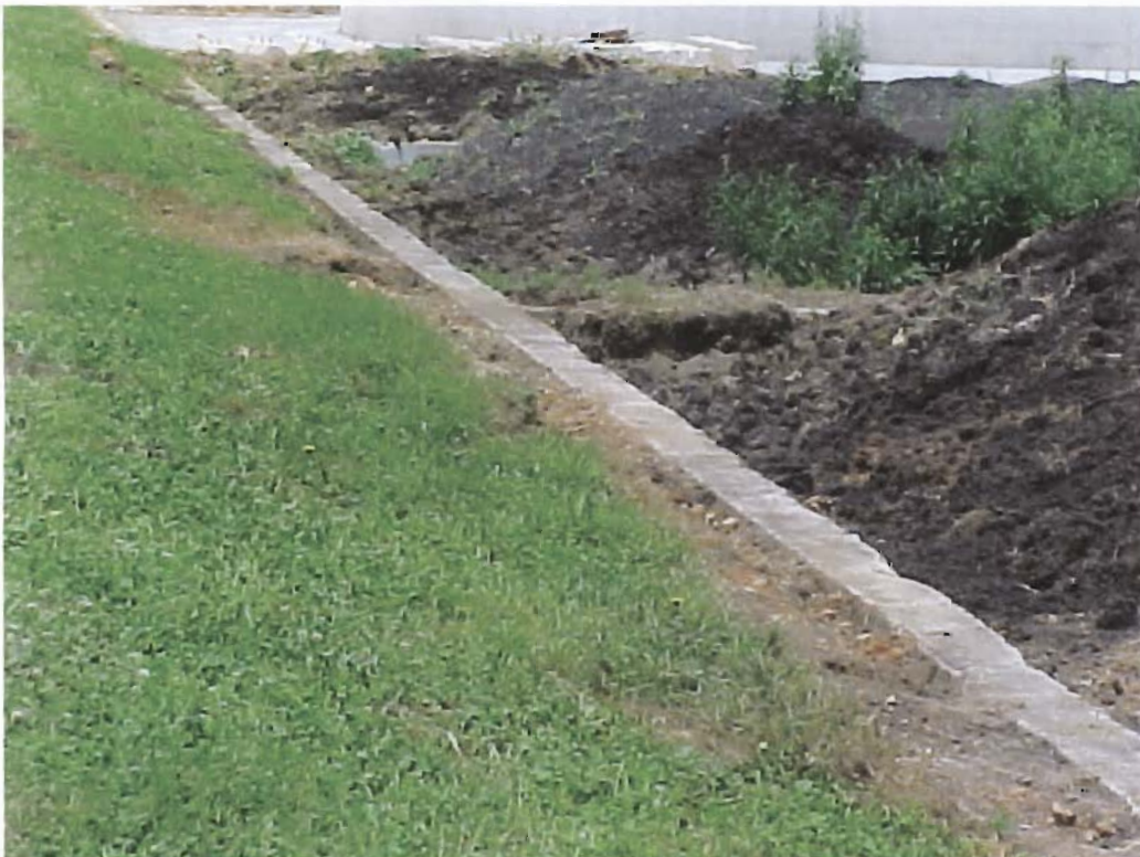
Figure # 2: Looking west on the south side of the sludge storage beds
