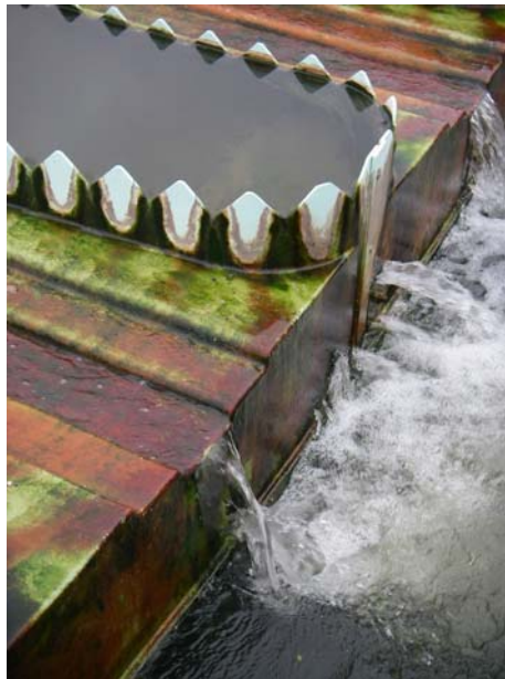
The above photo shows the leaking mounting bracket caps on the #2 final clarifier.
