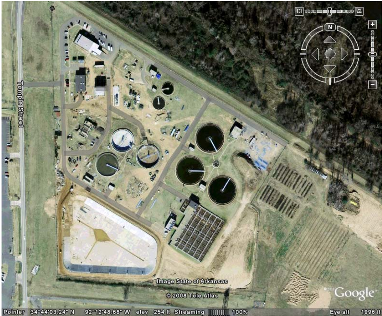
This photo shows the POTW in the spring of 2006. The large EQ basin on the bottom left went into service in July 2006.
