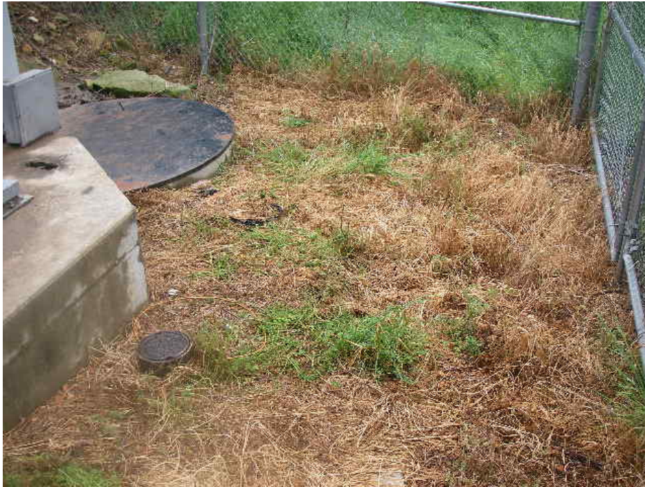
Lift station which failed
