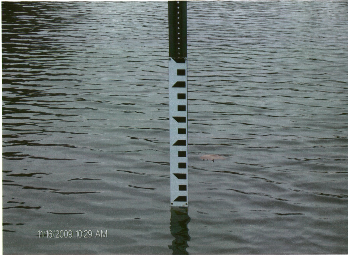
Image of Staff Gauge in the Polishing Lagoon The large marks indicate 6" with the top of the gauge representing the height of the levee.
