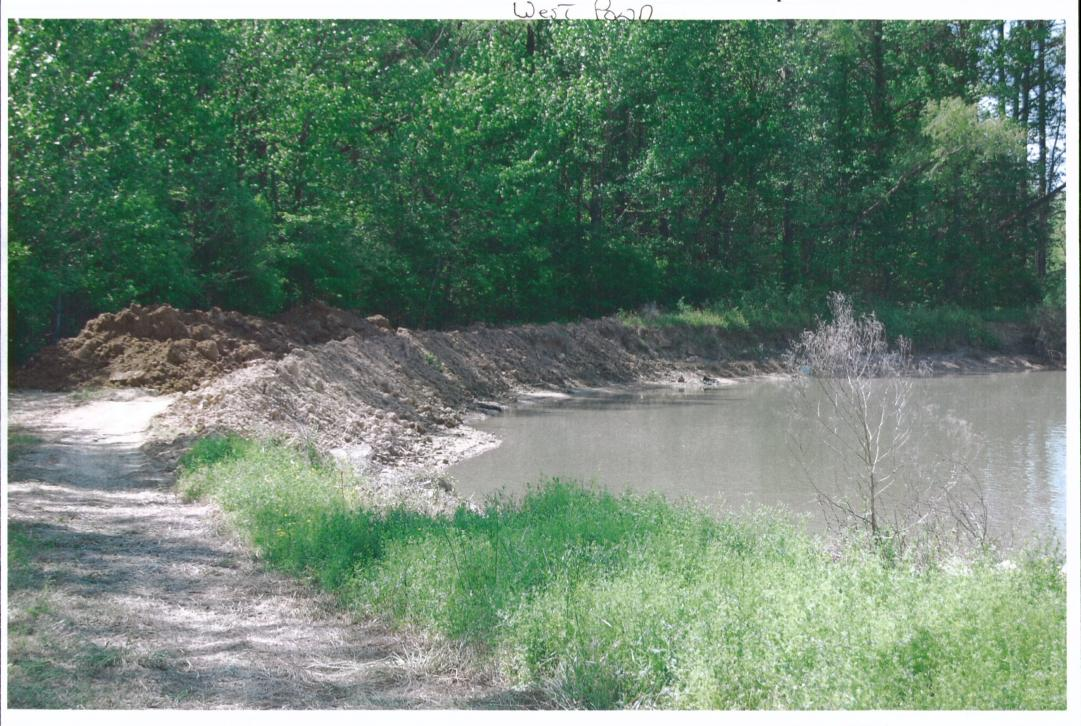
Uest Power Principal Finding #3/Facility has levees with excessive erosion. Picture shows dirt work being done on the levees to address the erosion problems
