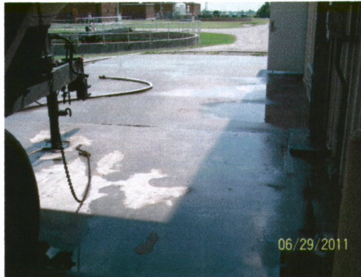
Cleaned loading area of bio-solids building
