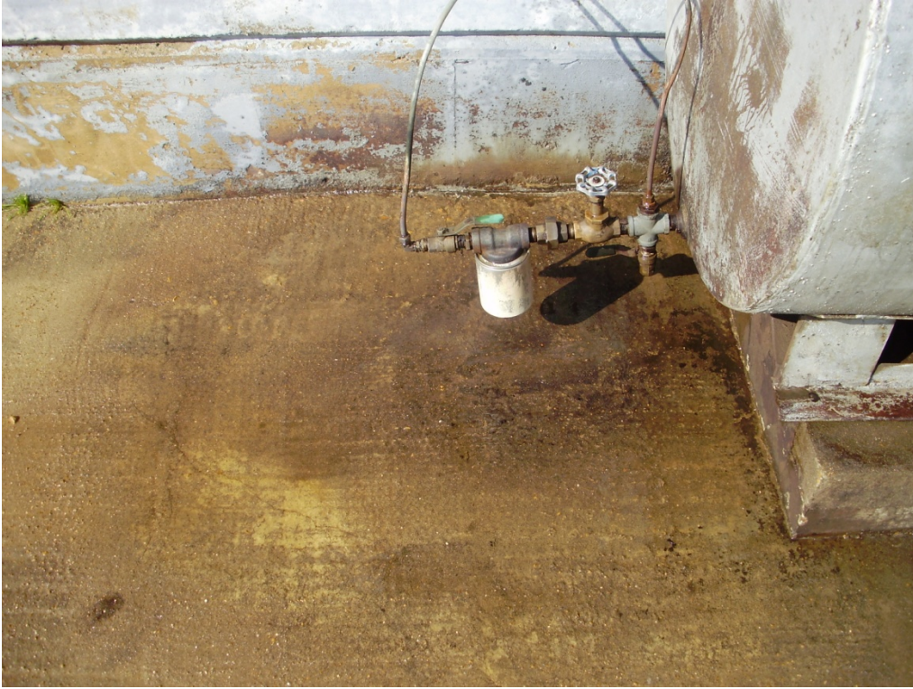
Area near diesel tank at Main Pump station after clean-up (above photo)
