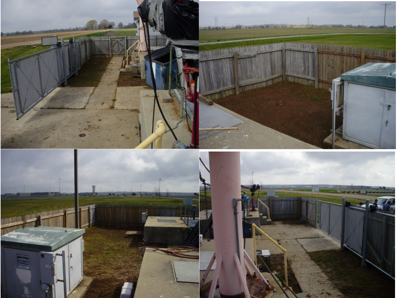
Ground inside fenced area at prison pump station after clean-up (4 photos above)
