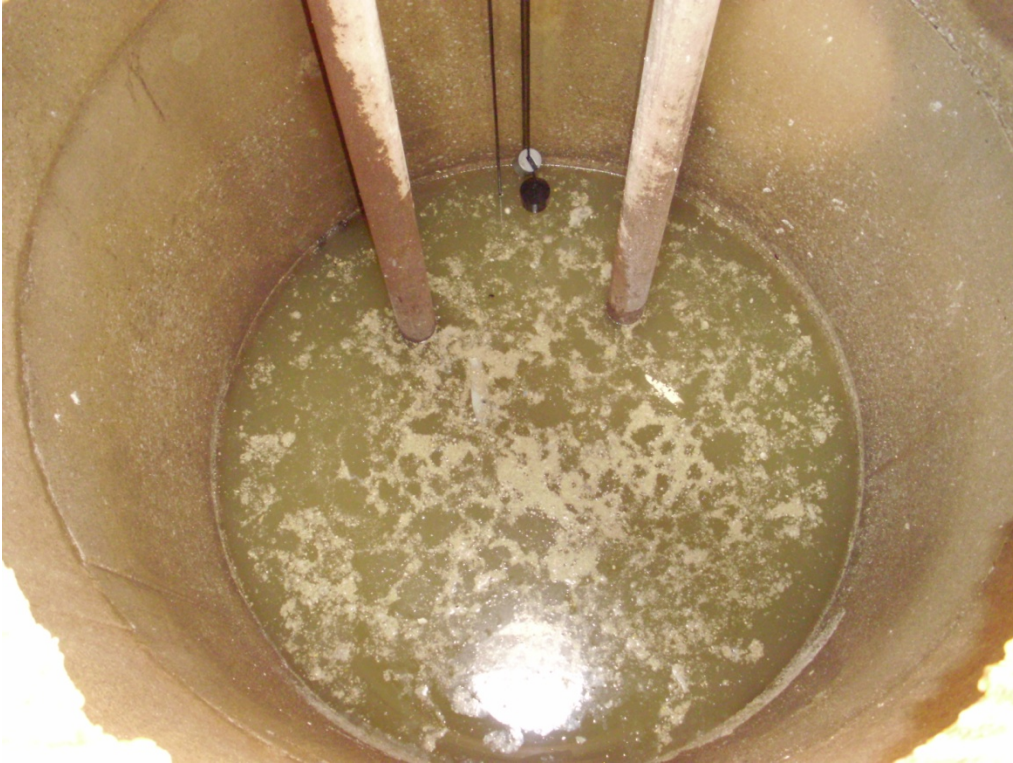
Wet well at Turner St. Lift Station after grease and solids removal. (above photo)
