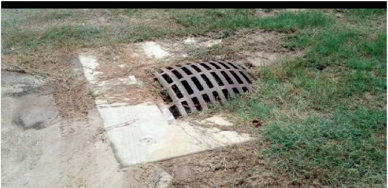
Concrete washout removal, Southwest side of property, Item #5, June 15, 2012
