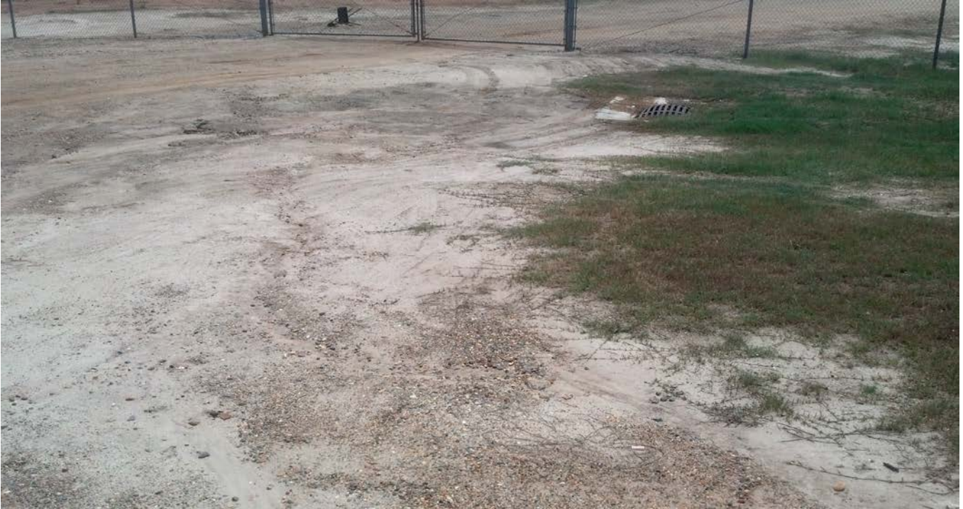
Concrete washout removal, Southwest side of property, Item #5, June 15, 2012
