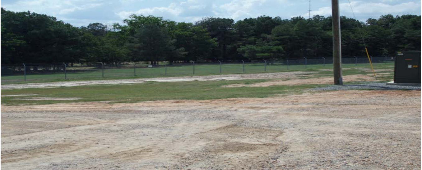
Concrete washout removal, Southwest side of property, Item #5, June 15, 2012
