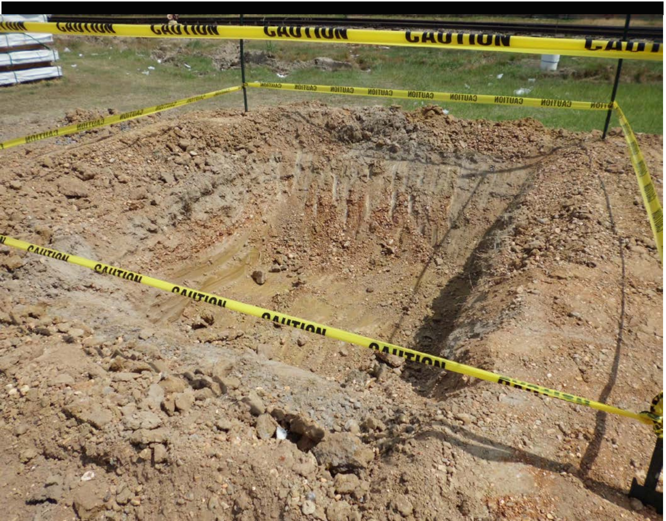
Designated Concrete Washout Area, June 15, 2012
