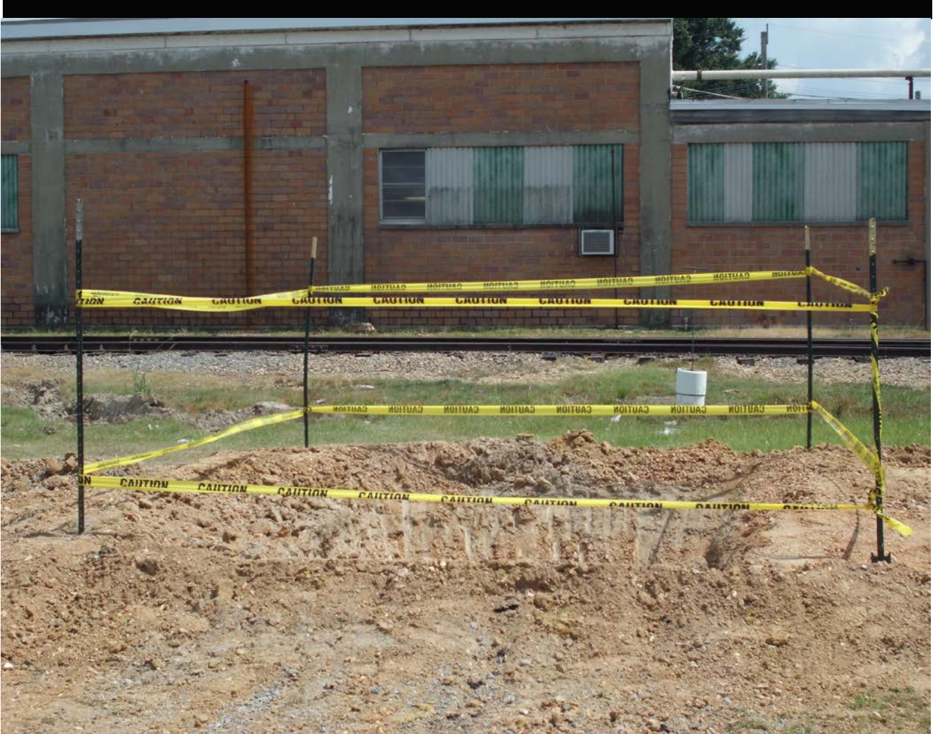
Designated Concrete Washout Area, June 15, 2012
