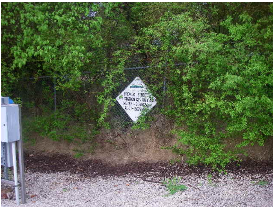
Brewer Street Lift Station signage
