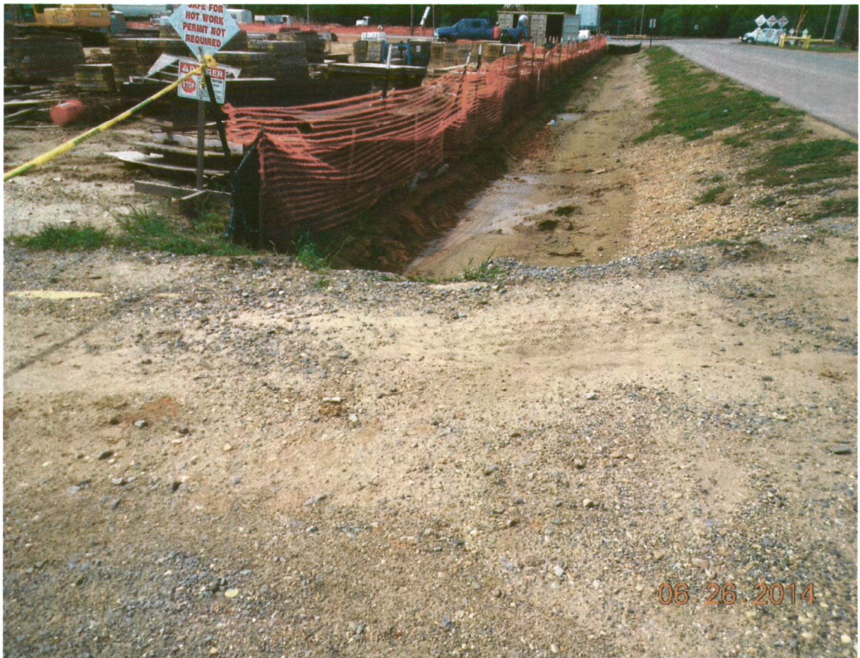
EDCC area referenced in ADEQ photo # 2. Silt fence has been removed along the ditch.
