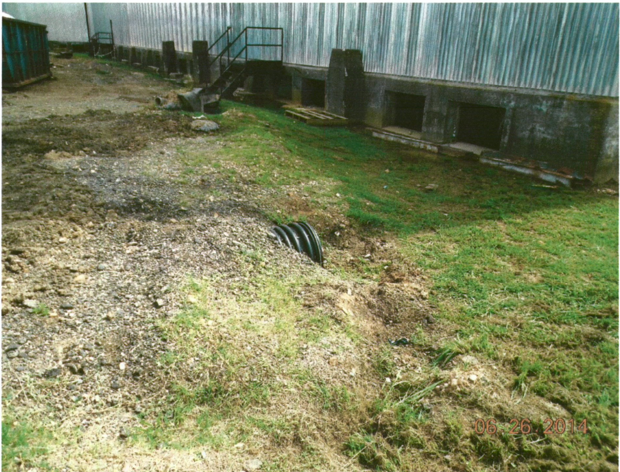
EDCC area referenced in ADEQ photo # 3. Silt fence has been removed.
