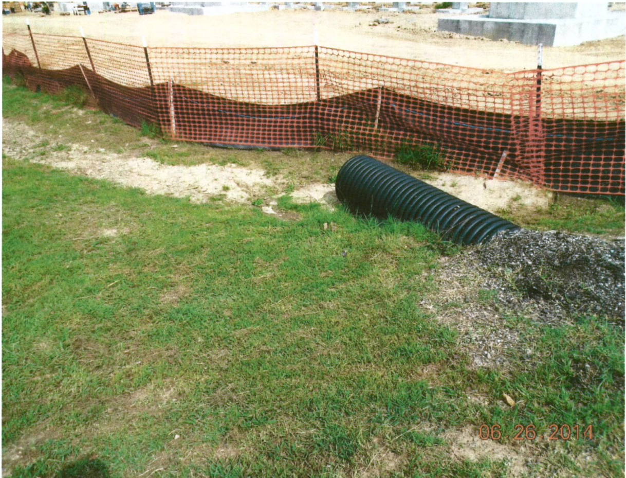
EDCC area referenced in ADEQ photo # 4. Silt fence has been removed.
