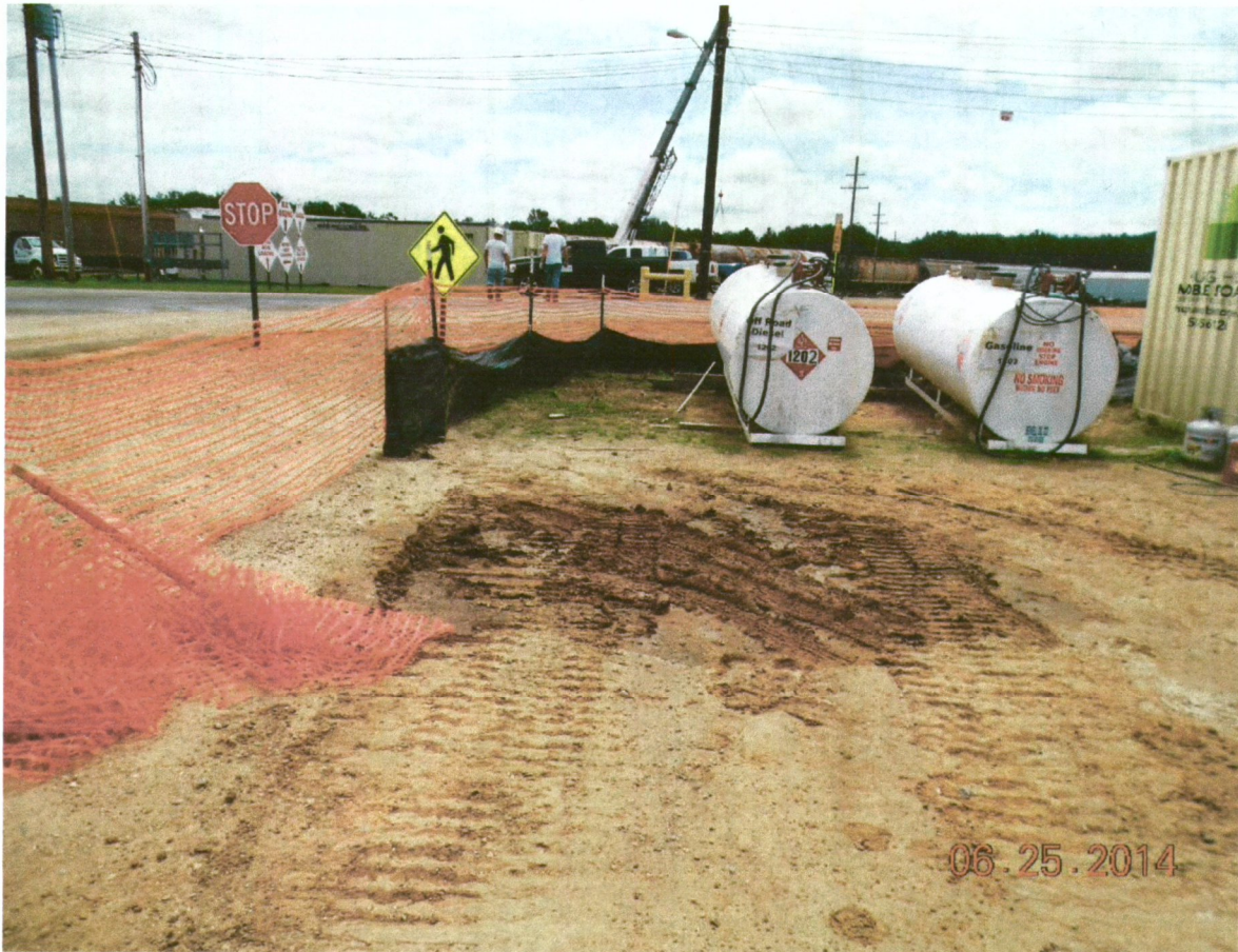
EDCC area referenced in ADEQ photo # 1. Silt fence has been repaired.
