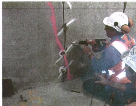
Drilling crack for installation of mechanical packers for polyurethane grout injection
