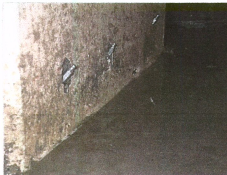
Mechanical packers installed
