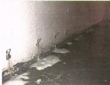
Hydroactive polyurethane grout installed
