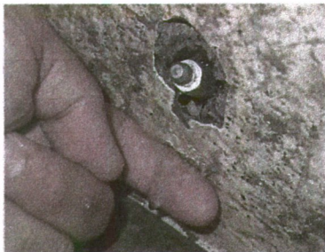
Installed packer
