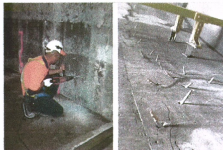
Drilling and installing packers along a crack line
